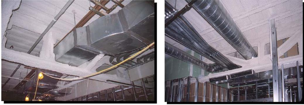
Figure 1.3: STMF with Piping and Duct Work
