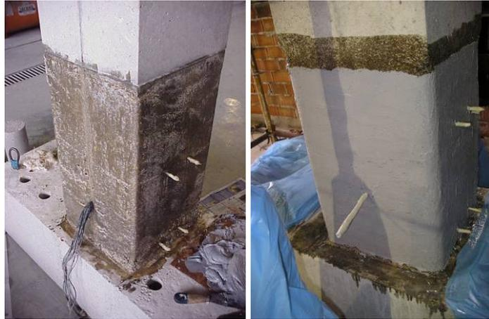
(a) Undercoat and epoxy mortar application for strengthened columns
