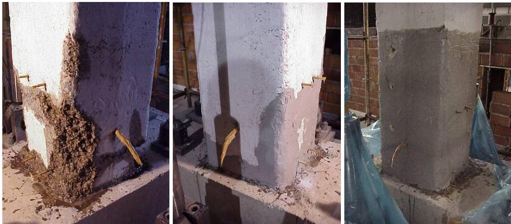
(b) Undercoat and epoxy mortar application for repaired columns after damage
