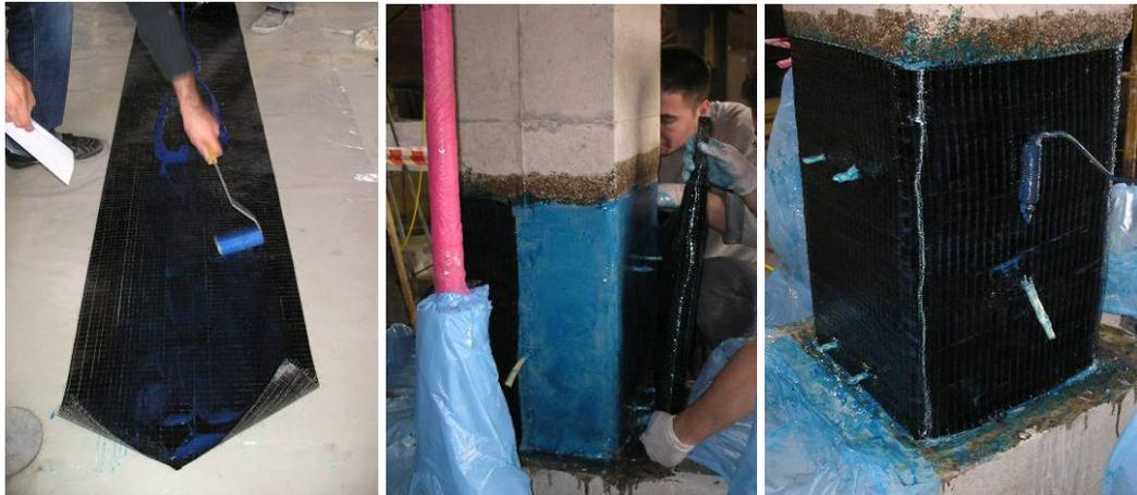
(c) CFRP wrapping
