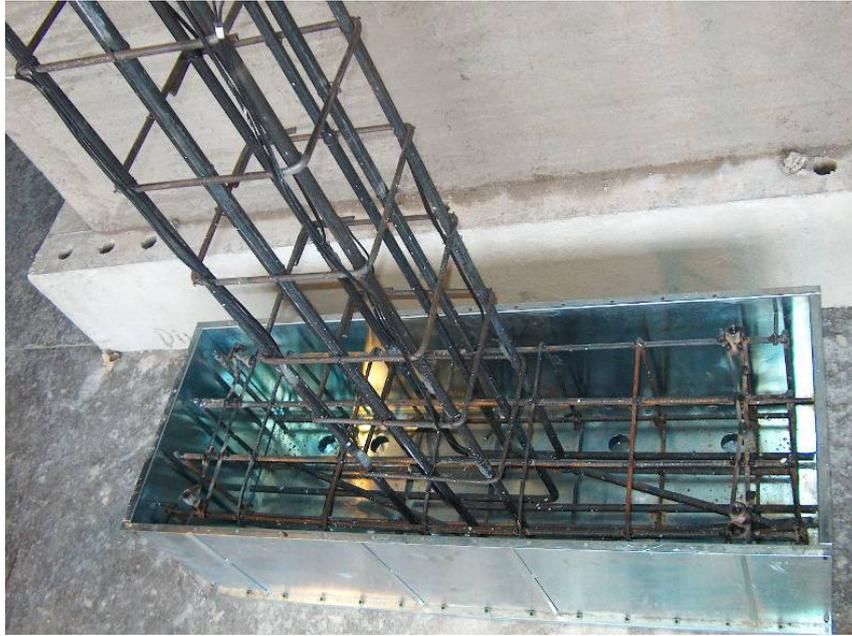
Figure 2.5 A typical footing formwork with reinforcement placed inside
