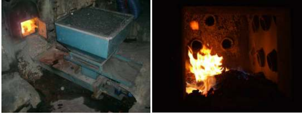
Figure 3.2 Views of the furnace in Şengül Hamamı (Source: Archives of the Author and Gülşen Dişli)
