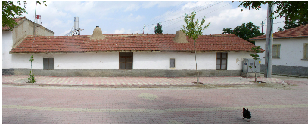
Figure XIV - A Hamit House. The earth composite roof is replaced with terracotta tiling but the chimneys are original. Windows are slightly modified in their size and the door from the Peç Üy, facing the street, is replaced a small window (source: Özüm İtez, 2008)
