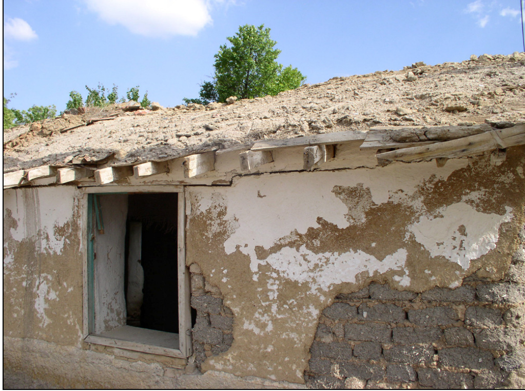
Figure XIII - A close-up look to the earth composite roof and adobe wall of a ruined Hamit House. (source: Özüm İtez, 2008)
