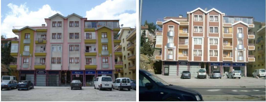
Figure 3.1 The improvement of the frontage of the buildings in terms of harmony
