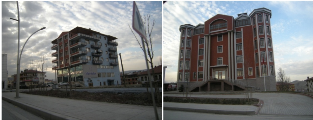
Figure 2.14 A view of buildings without proximity to others
