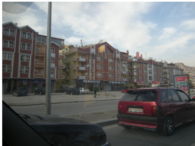
Figure 1.10 View of the cladding and side elevation from a moving vehicle
