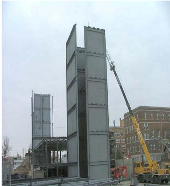
Figure 1.7 – Core Wall in the Middle of ING Building, Montreal, CANADA [23]
