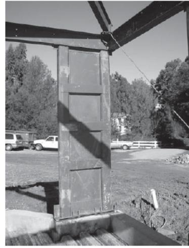
Figure 1.4 – Residential Building With SPSW System in Atherton, CA [23]
