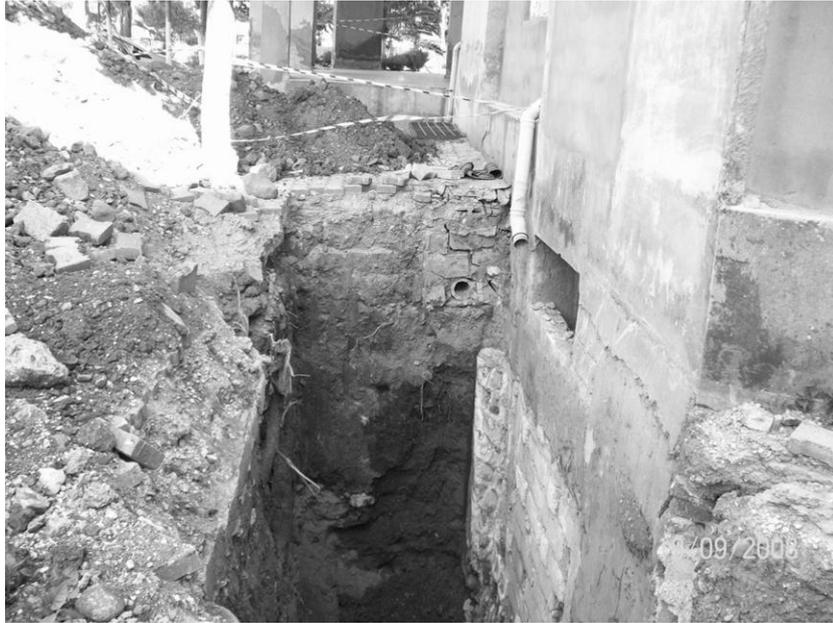
Figure D.4: Foundation excavation for eccentric reinforced concrete shearwalls
