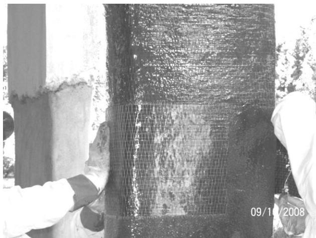
Figure D.2: Column repaired against corrosion.
