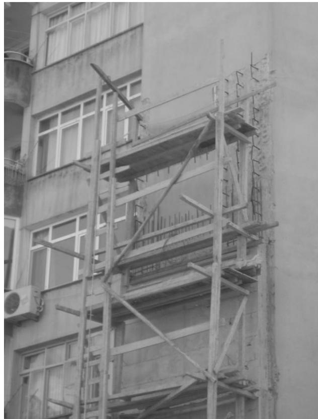
Figure D.5: Production of eccentric reinforced concrete shearwalls.
