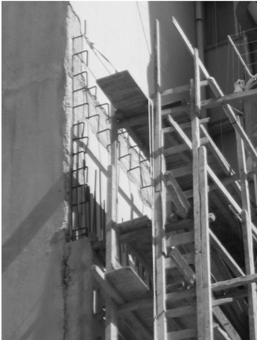
Figure D.6: Production of eccentric reinforced concrete shearwalls.
