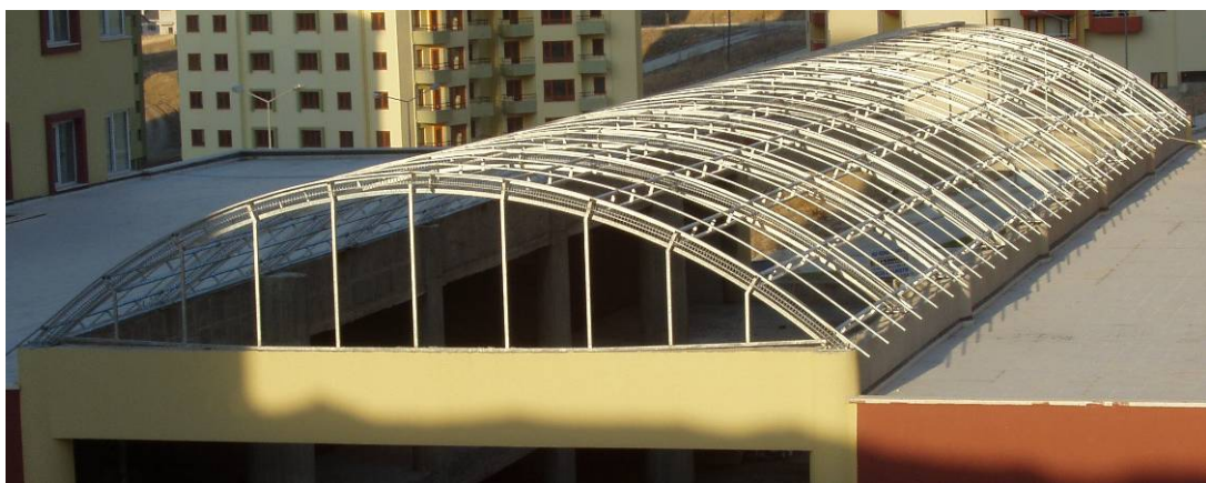
Figure 3 Helical wire core truss member used in roof construction.
