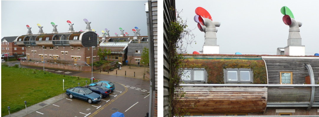
Figure 3.18 and Figure 3.19: BedZed Ventilation strategy: Heat-recovery moving wind cowls
