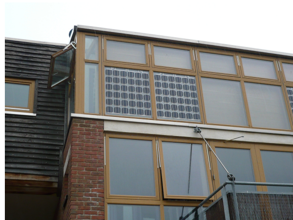
Figure 3.14: PV cells on the windows
