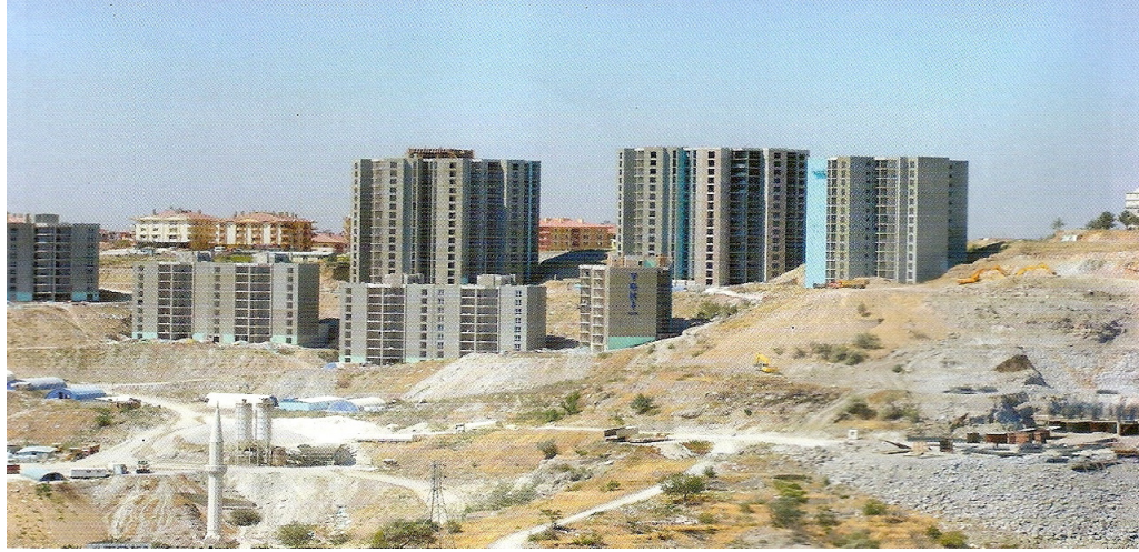
Figure 50 Constructed Buildings for Right owners
