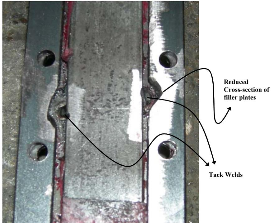
**Figure 2.16 – Photo of Tack Weld Attachment for Encasing Member**
