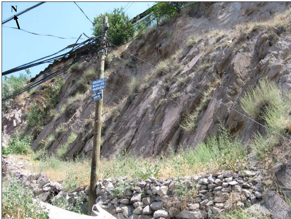
Figure 2.25 The flow structures of andesites located on the upper parts of the hill near B-1 and BH-2.
