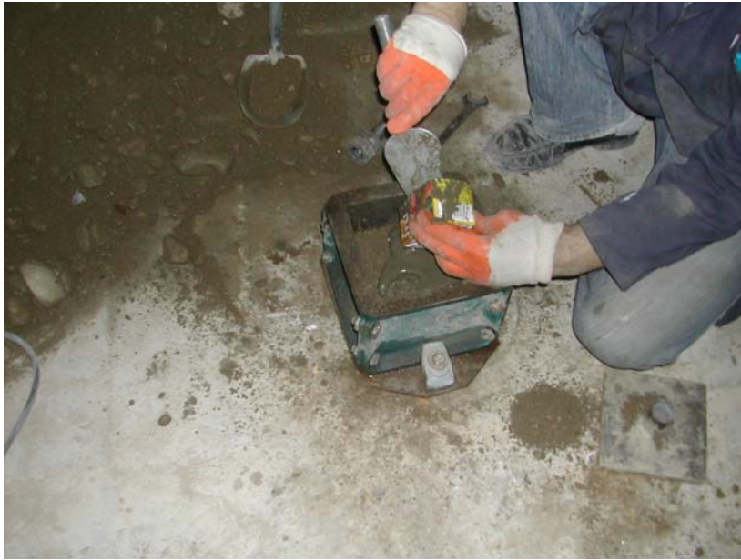
Figure 3.10 A view of the application of bedding mix
