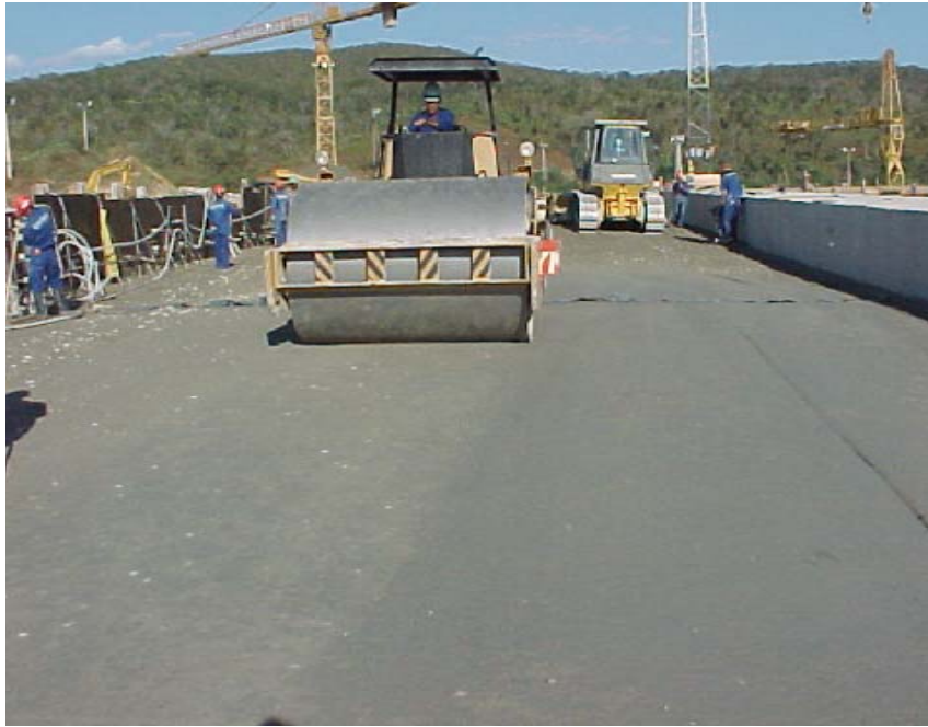
Figure 2.3 A view of compaction of concrete using vibrating roller
