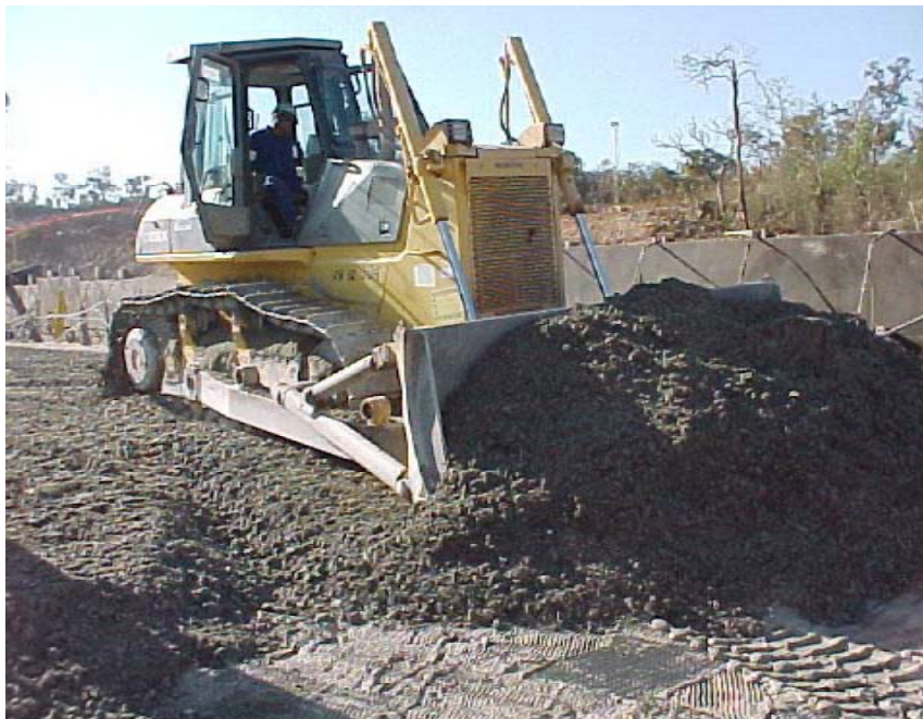
Figure 2.2 A view of spreading of RCC layers
