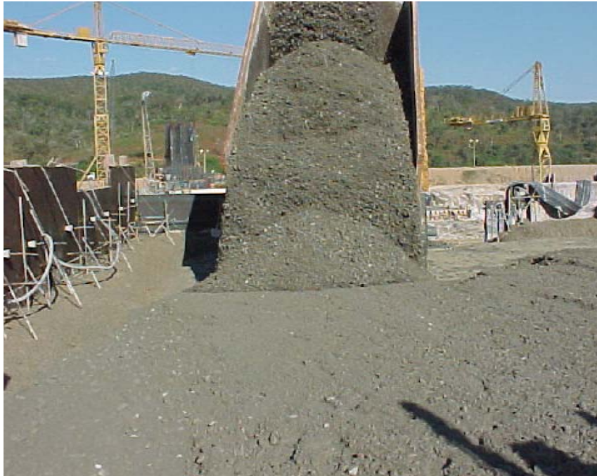
Figure 2.1 A view of transportation and dumping of concrete
