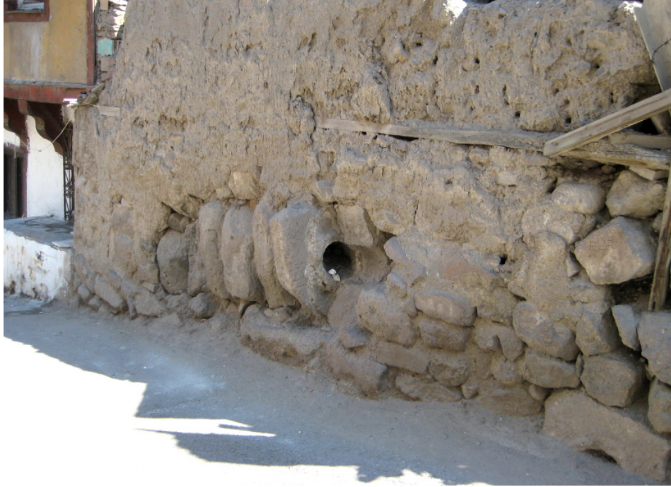
Figure 9: Block course opposite Saraçsinan Mescidi at Atpazarı Sokak (Photo: Emre Kaytan).
