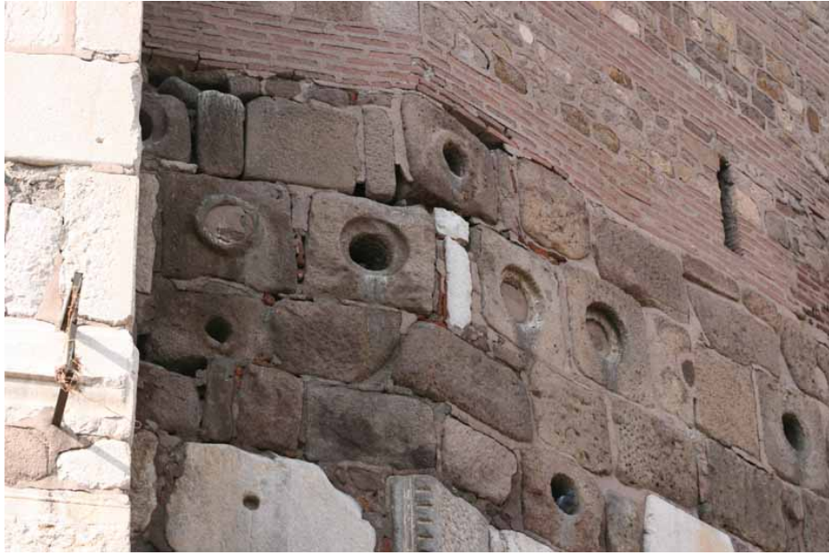
Figure 27: Re-used pierced blocks on the walls of the city citadel (Photo: Emre Kaytan).
