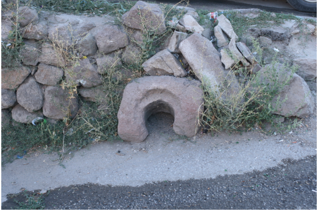
Figure 13: Scattered pierced blocks at Atpazarı Sokak (Photo: Emre Kaytan).
