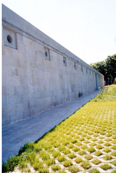
Figure 22: Exterior view, “Boşlukta Beyaz Ev”, 1997, Nevzat Sayın; Saray, Tekirdağ, Turkey.
