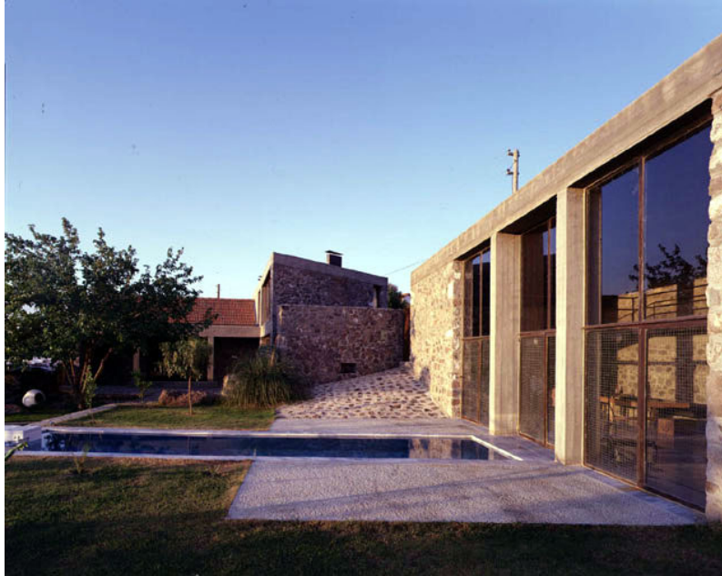
Figure 27: View north; pool and glazing on the west façade, Senan House, Nevzat Sayın, Dikili, İzmir Source: http://archnet.org/library/images/one-image-large.jsp?location_id=5656&image_id=19352 (accessed on 18.08.2008)
