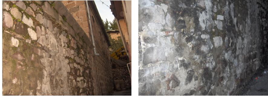
Figure 4.4 Views of biological growth as active deterioration zones together with white staining and/ or salt deposition & material loss in relation with cement repointing on surfaces of the south façade of the building.
