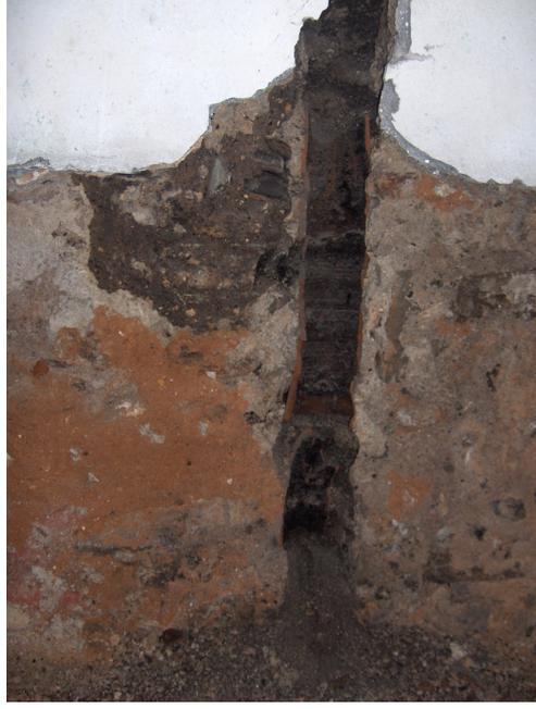
Figure 2.12 A view of *tüteklik* rising inside the wall up to the roof in Yıldırım Beyazıt Hamamı, in Mudurnu, Bolu.
