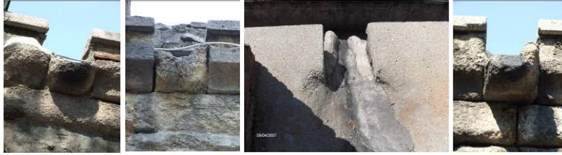
Figure 4.15 Views of the spouts, WS1, WS4, WS5 and WS7 (from left to right, respectively) showing the severely deteriorated sluiceways due to cement-based mortar repairs.
