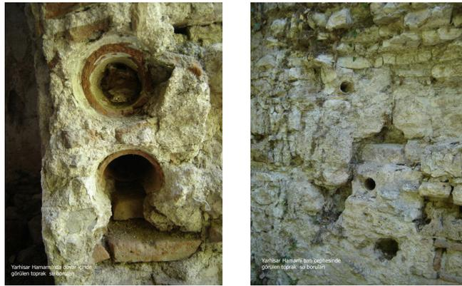
Figure 2.19 Terracotta pipes arranged in two rows on top of each other carrying hot and cold water Yarhisar Köyü Hamamı, in Bursa.
