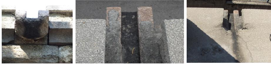
Figure 4.11 The front and top views of the original water spout, WS6, having flow dimensions of 10cm x 7cm in width to depth, respectively.
