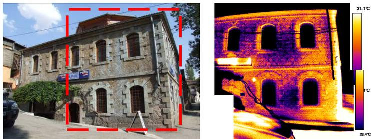
Figure 4.8 The infrared image of the selected region at the north façade, showing the severe material loss as warmer areas and the detachments which were not observed visually as colder areas, both suffering from the roof drainage faults.
