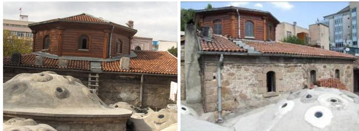
Figure 3.9 Views of the pitched roof, A1, over the frigidarium of women's part (at left) and the pitched roof, A2, over the frigidarium of men's part (at right) with their discharge components: gutters and downpipes *Source: Archives of the Author.*
