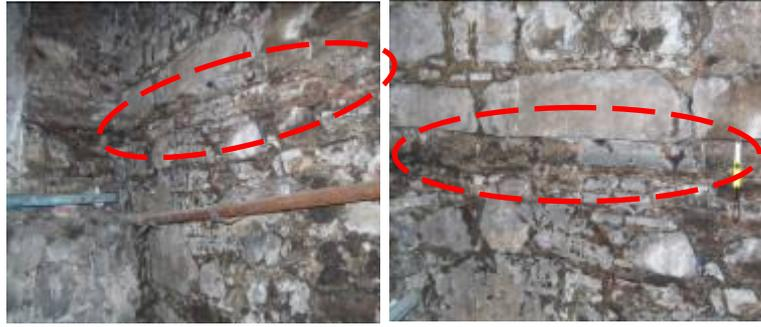
Figure 3.4 Views of the traces of the historical terracotta piping in Şengül Hamamı, running at the west wall of the firewood storage room.
