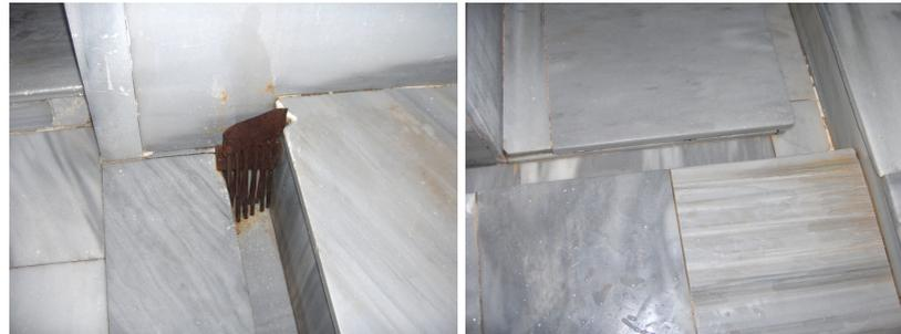
Figure 3.7 Views of waste water channels and of floor drains in Şengül Hamamı.
