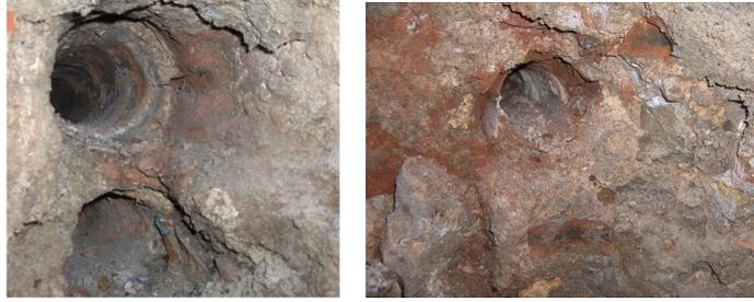
Figure 2.18 Terraces of terracotta pipes observable as the horizontal bant on the wall of Yıldırım Beyazıt Hamamı in Mudurnu, Bolu.
