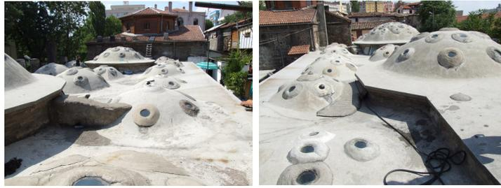
Figure 3.8 General views of the mesh-reinforced concrete roof above the caldarium and tepidarium sections.
