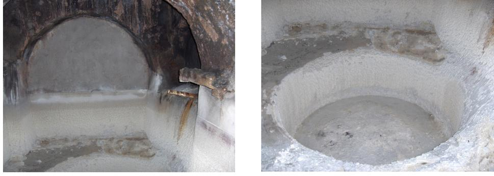
Figure 2.2 A view of the water storage room with brick barrel vault covering above and concave boiler below in Yıldırım Beyazıt Hamamı in Mudurnu, Bolu.
