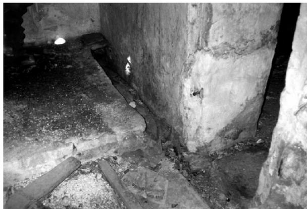
Figure 2.31 A view of waste water collection and discharge channels in Özbek Hamamı, in Urla, İzmir.
