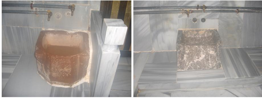
Figure 3.5 Views of the stoppers belonging to the old water supply system located close to the level of present piping system.
