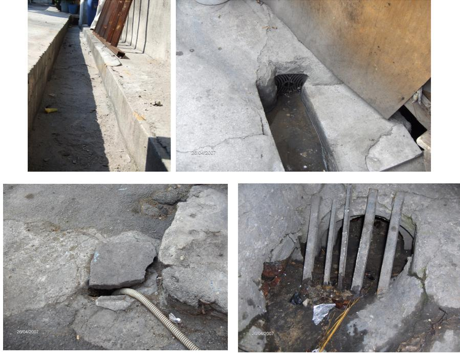
Figure 3.12 Views of the interior gutter and the drain discharging water from concrete clad flat roof, B2 and view of the drain line (buried in the garden) towards the drainage network (buried under the street).
