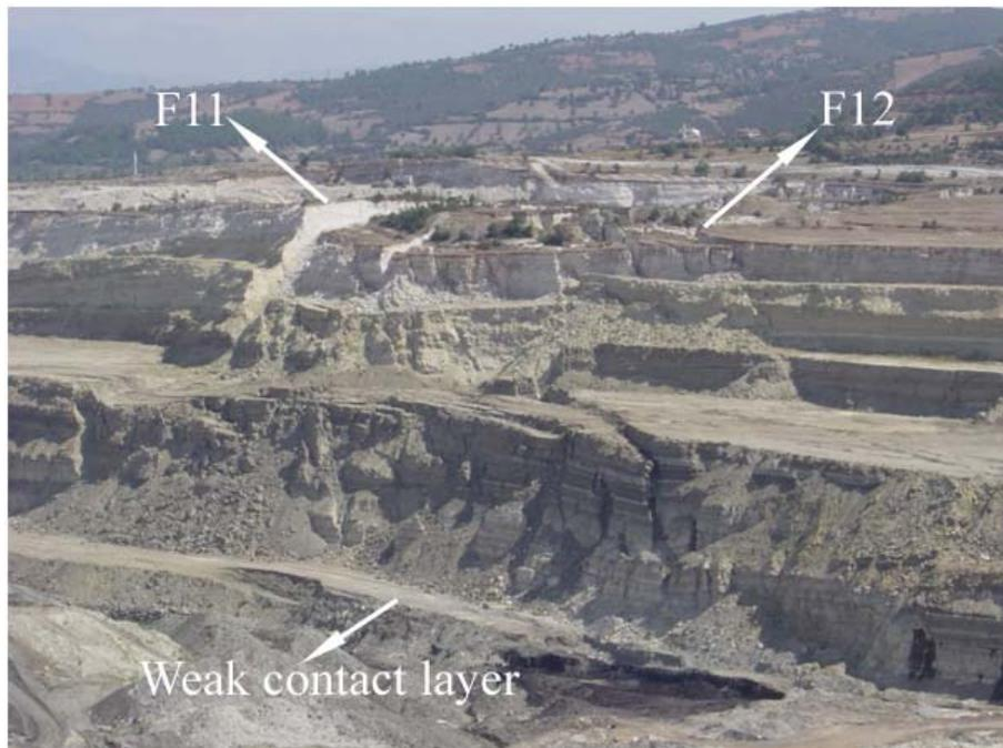
Figure 5.10 Orhaneli A-6 panel slope failure
