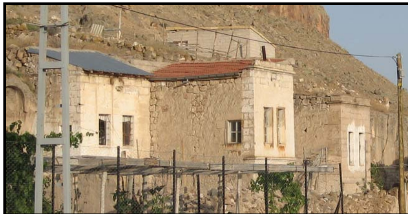
Figure 4.37. The directions of the roof slope and its material are different in these two houses.
