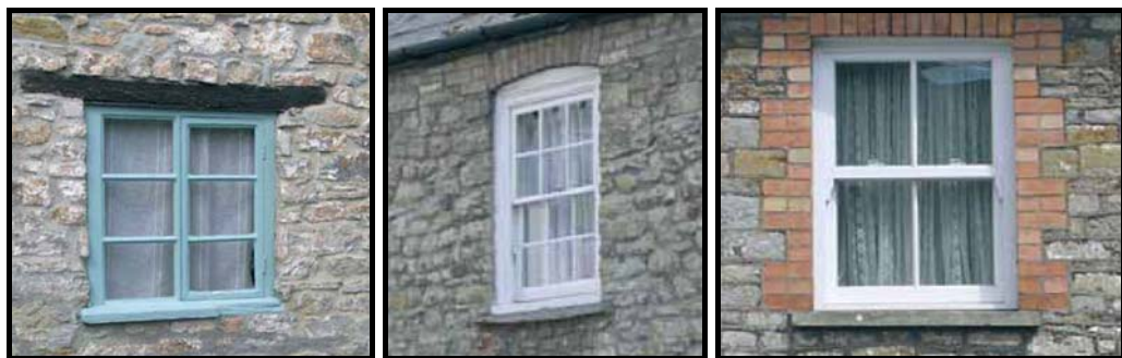
Figure 2.8 a) Timber lintel, b) Stone/brick arches over windows and stone/timber sills, c) Windows with brick detailing.
