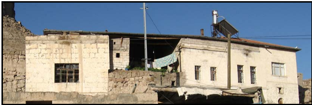
Figure 4.36. Flat roofs replaced with a single hipped roof to cover five houses.
