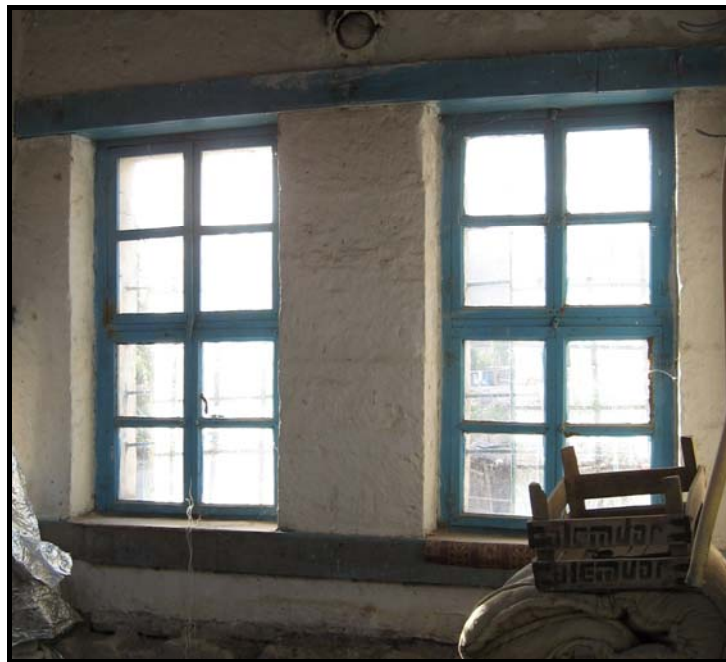
Figure4.19. Typical side hung casement timber frame window.
