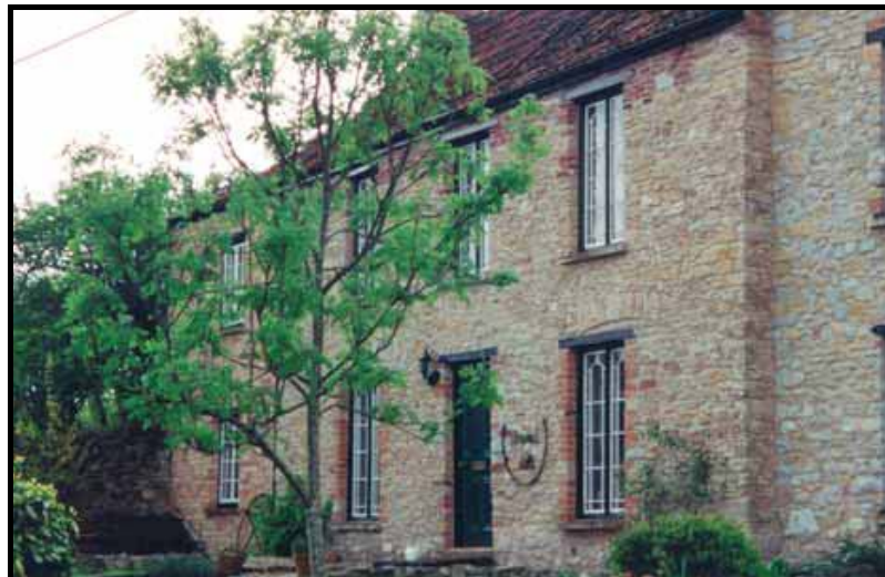
Figure 2.9. A feature of Wedmore, England is the use of local Wedmore stone as a building material for houses.
