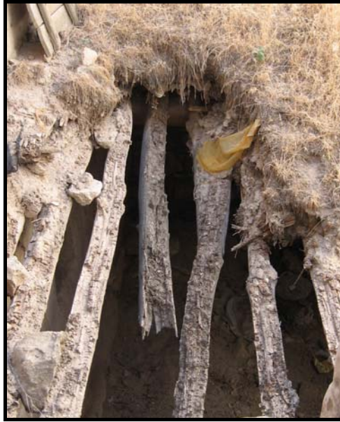
Figure 4.27. The materials used to construct a traditional flat roof are timber beams, branches and compacted earth.
