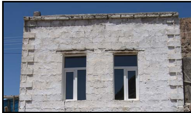
Figure 4.34. Photo showing the replacement of original timber window frames with PVC ones.
