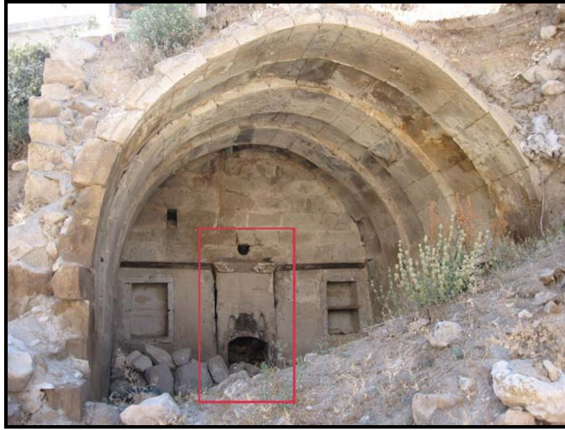
Figure 4.24. The hearth which was on the ground floor failed to heat the first floor.
