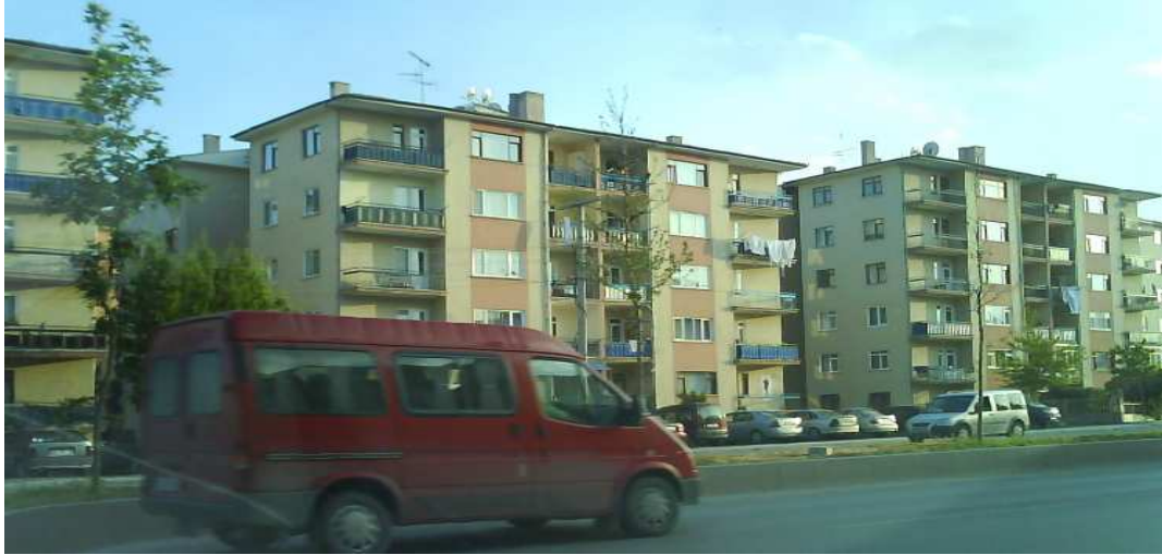
Figure 6.63: Houses produced by housing cooperatives from Selçuklu Quarter
