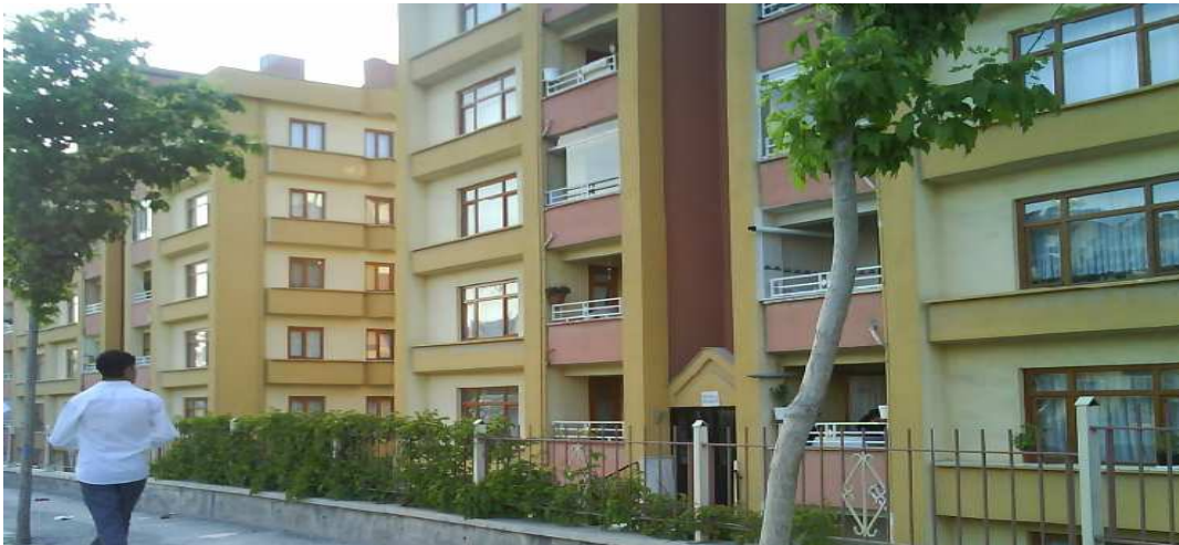
Figure 6.62: Houses produced by housing cooperatives from Selçuklu Quarter
