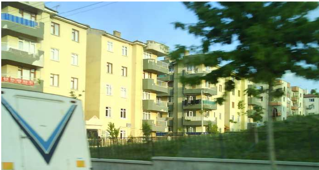
Figure 6.54: Housing types produced by housing cooperatives in the Andiçen Quarter
