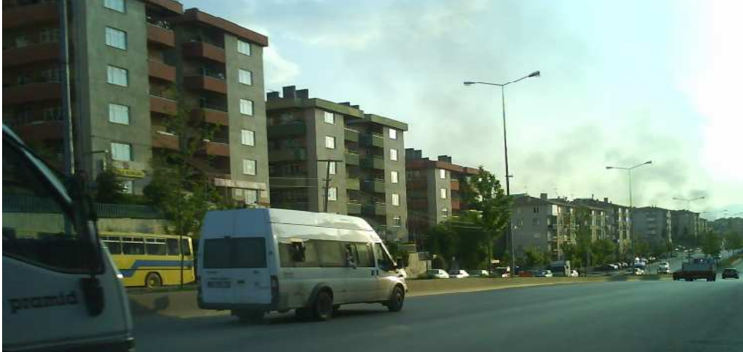
Figure 6.61: Houses produced by housing cooperatives from Selçuklu Quarter
