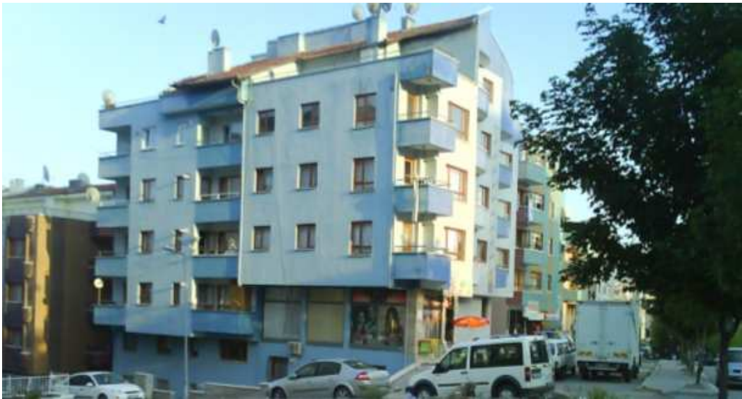
Figure 6.27: Yap-satci housing provision from Atakent
