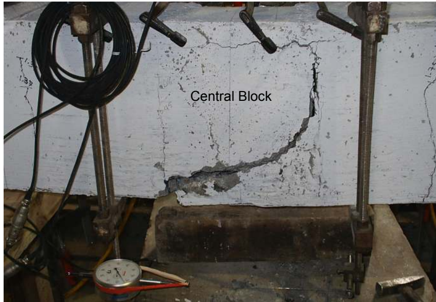
Figure 3.21(a) Crack pattern of specimen B2 after failure
