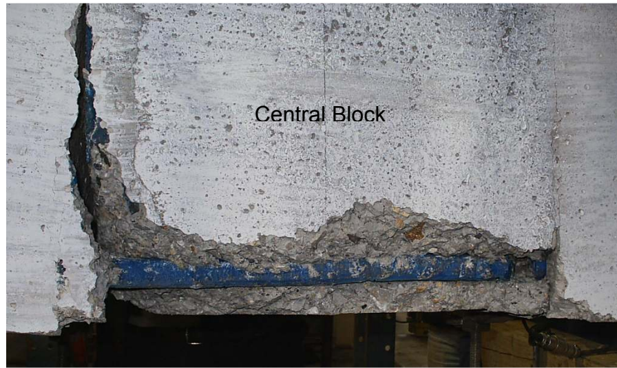
Figure 3.24 Specimen B3 after failure (combined cone and splitting)
