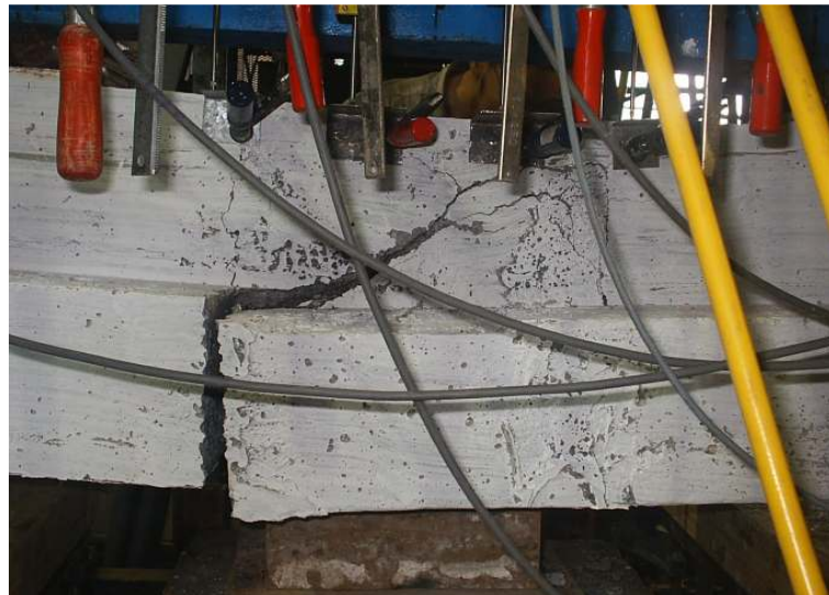
Figure 3.27 Specimen C3 after failure (combined cone and splitting)
