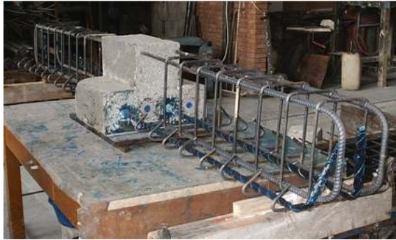
Figure 2.8 Specimen C3 of series C before casting outer blocks
