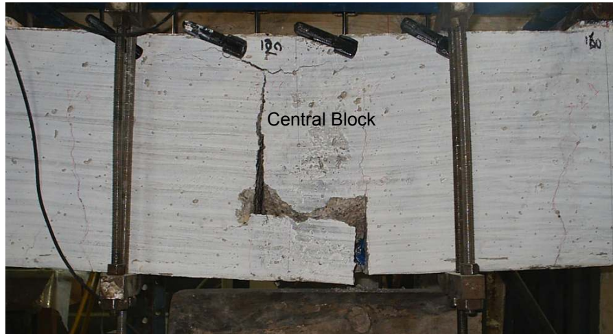
Figure 3.18(a) Crack pattern of specimen B1 after failure
