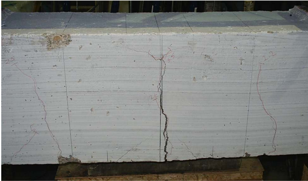
Figure 3.12 Crack pattern of A2 after failure
