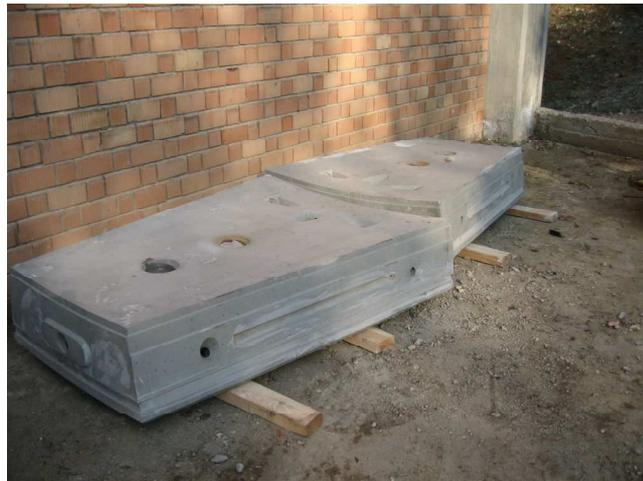
Figure 3.1 Precast TBM Key Segments
