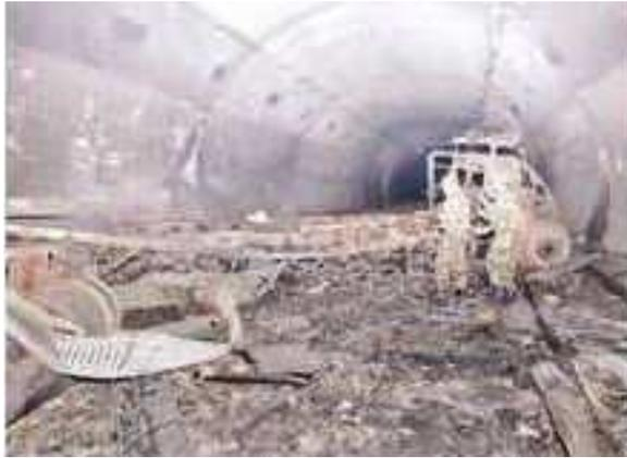
Figure 2.1 Large Extreme Tunnel Fire (Trucks Carrying Missiles Caught Fire and Melted, No Signs of Concrete Spalling),
