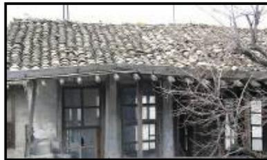
**Figure 71:** The Missing Roof Tiles at the Edges of the Eaves (author April, 2003)
