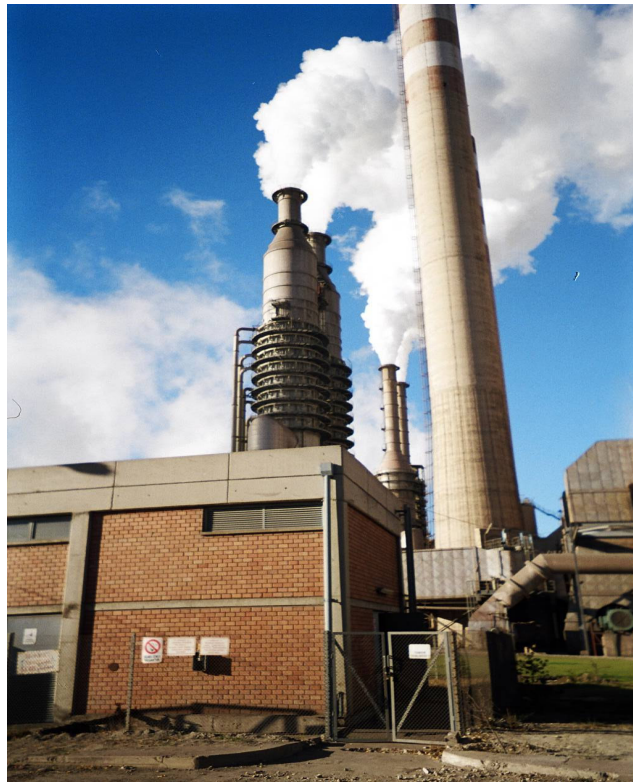
Figure 2.12 Stacks of the FGD systems at Çayırhan Thermal Power Plant
