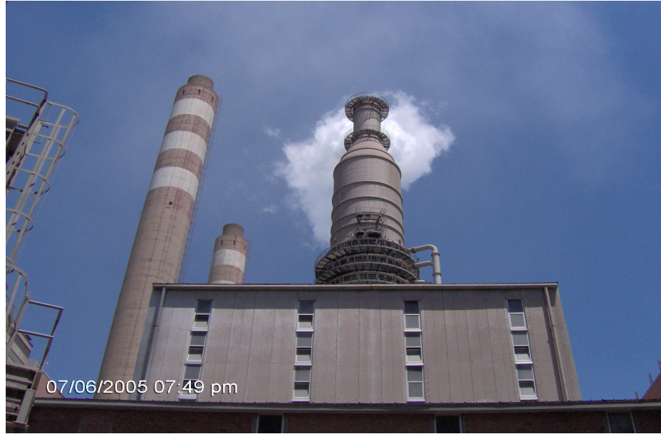
Figure 2.11 Stacks of the FGD systems at Çayırhan Thermal Power Plant
