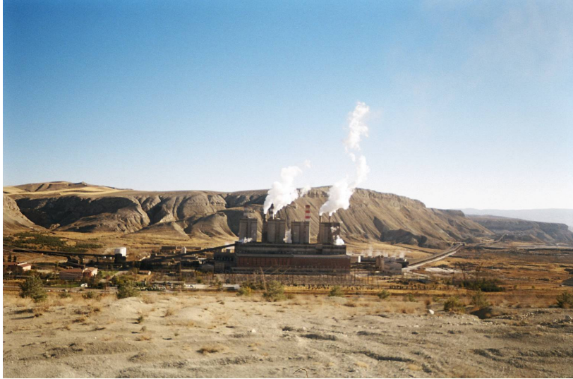
Figure 2.2 General view of the Çayırhan Thermal Power Plant
