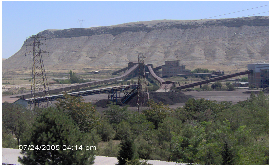
Figure 2.7 Coal transportation systems in Çayırhan Thermal Power Plant
