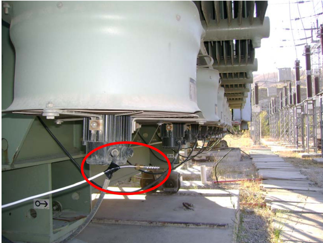
Figure 5 Resistive Thermometer of Ambient Temperature installed in the field
