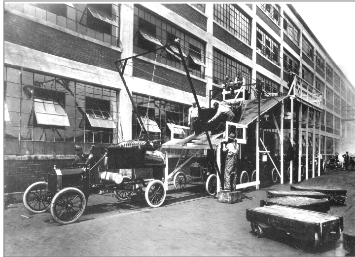
Figure 8: Chassis assembly of Ford Model T, Highland Park Factory, 1915 (Source: http://www.biz.colostate.edu )
