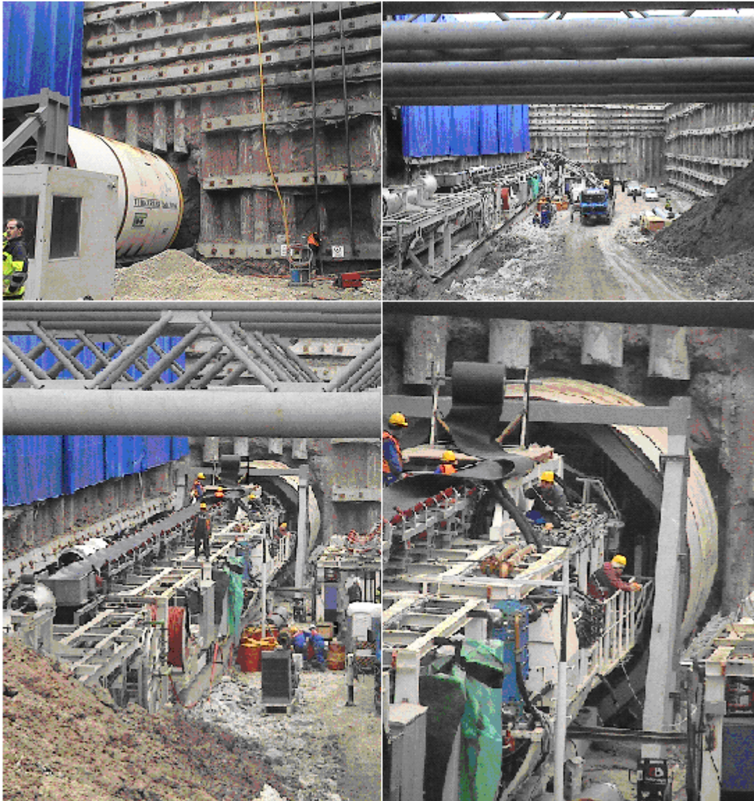
Figure 1.13. TBM implementation and portal site of the Keçiören – Tandoğan metro alignment
