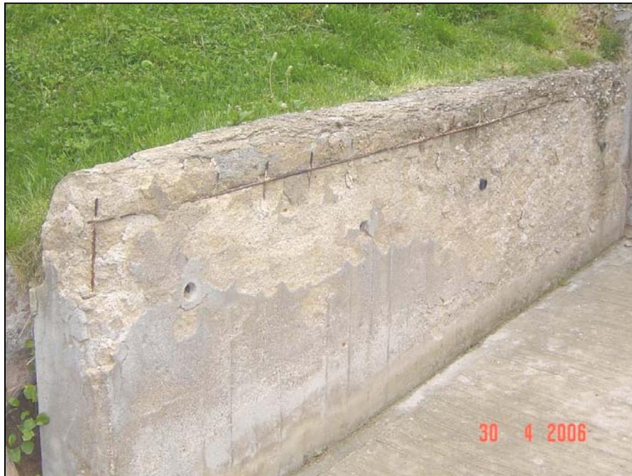
**Figure 3.12: A typical example of deterioration in concrete due to freezing and thawing**
