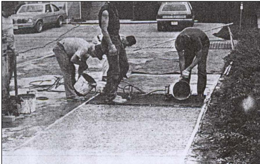
**2.28: Infiltration of the steel fiber bed with the slurry in pavement overlay application [31]**
