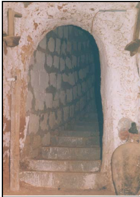
Figure 4.29 View of the staircase from the courtyard.
