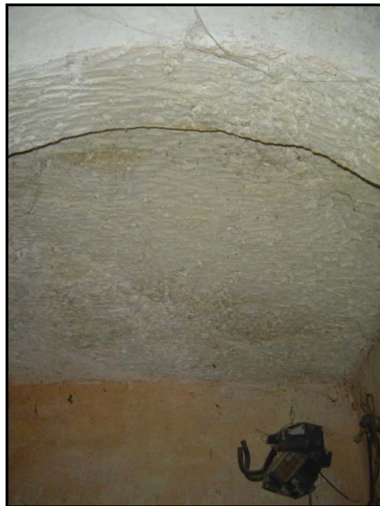
Figure 4.27 Barrel vaulted ceiling of troglodyte.
