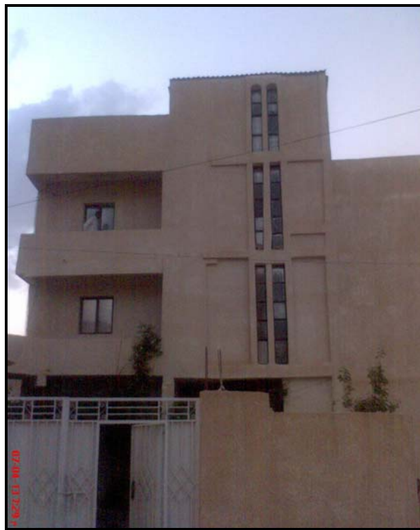
Figure 4.34 General view of the contemporary house in Gharyan.
