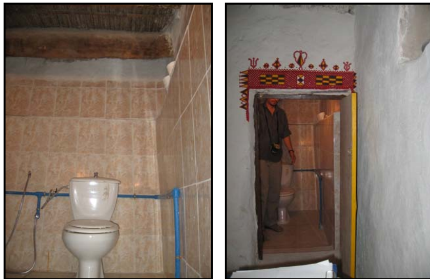
Figure 4.48 Contemporary W.C. and the ceramic walls in the traditional house of Ghadames.
