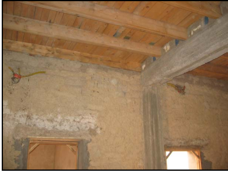
Figure 4.5 Reinforced concrete skeletons of the houses in Tuneen.
