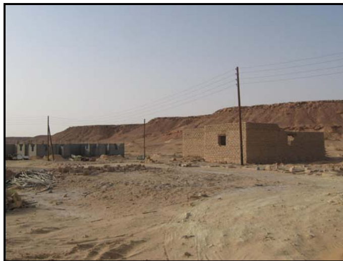
Figure 4.4 A general view of houses under-construction in Tuneen.
