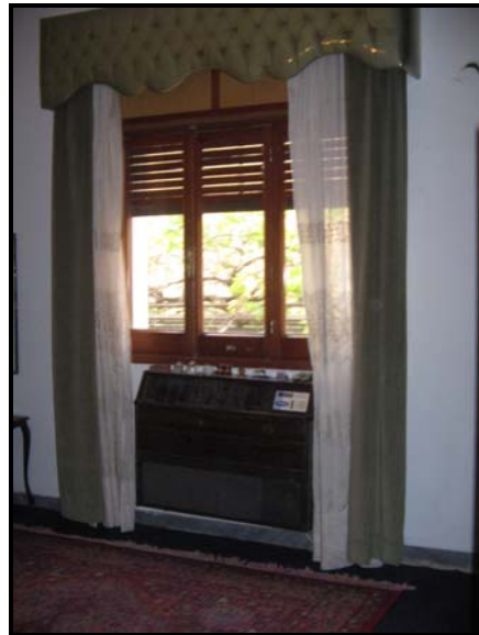
Figure 4.21 Air-conditioning system of the contemporary house in Tripoli.
