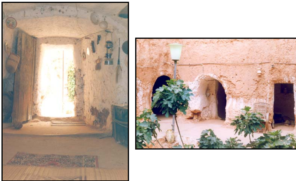
Figure 4.25: The entrance of the room viewed from inside and from the courtyard.
