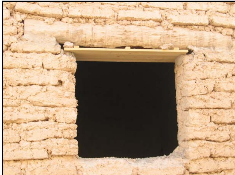
Figure 4.8 Wooden lintels over a window opening for a house in Tunes.
