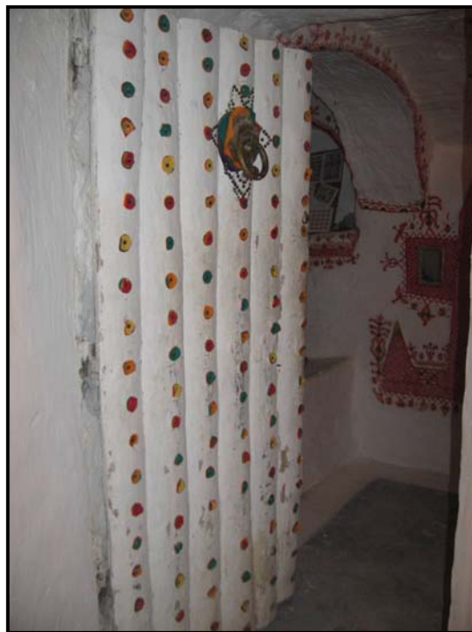
Figure 4.44 Wooden door of the traditional house in Ghadames.
