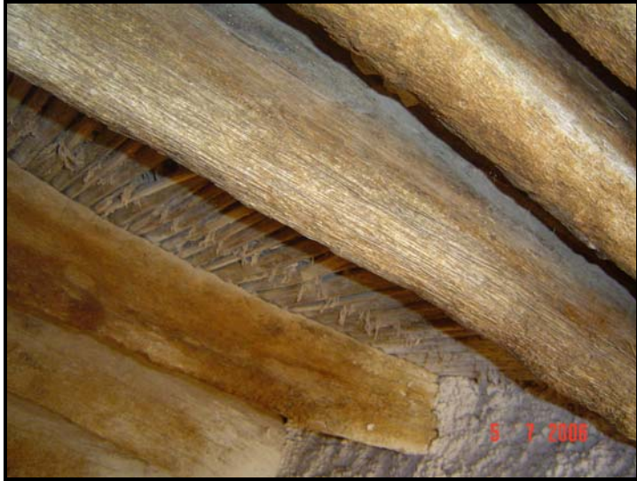
Figure 4.43 Palm wood beams used for supporting the ceiling of the traditional house in Ghadames.
