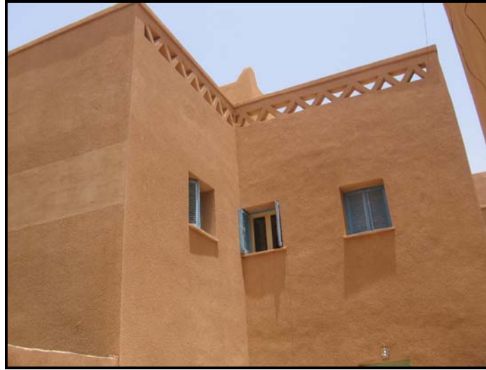
Figure 4.53 Windows of the contemporary house in Ghadames.
