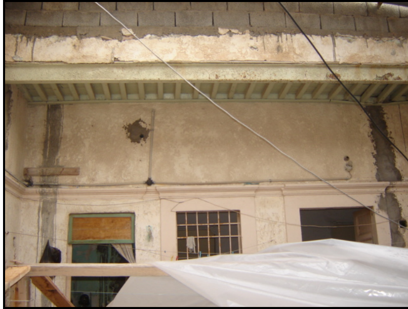
Figure 4.15 Concrete block and cement plaster used for repair work in the traditional house in Tripoli.
