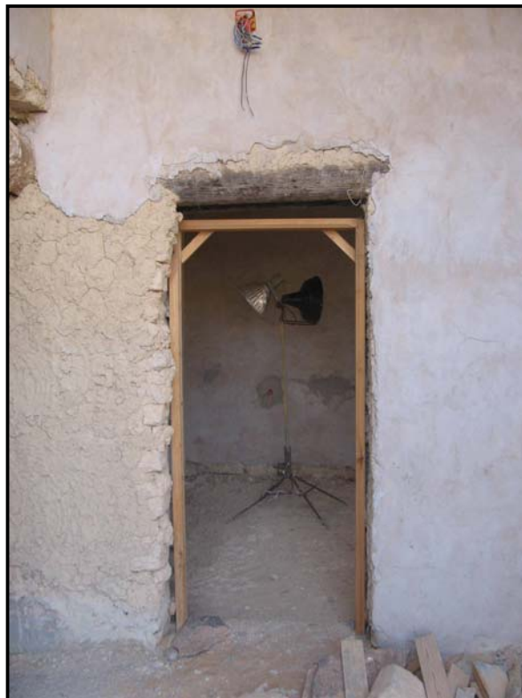
Figure 4.10 Plastering with mortar of the houses in Tuncen.
