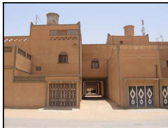
Figure 2.27b A general view from the new city of Ghadames, showing the adapted features of the old city "the connected roofs".
