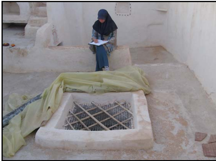
(a) Opening at the roof (top view)
