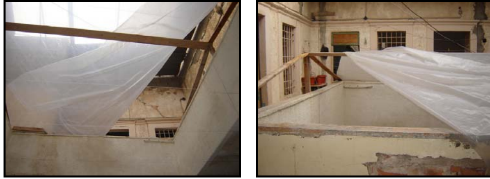
Figure 4.12 Temporary plastic sheets covering the courtyard.
