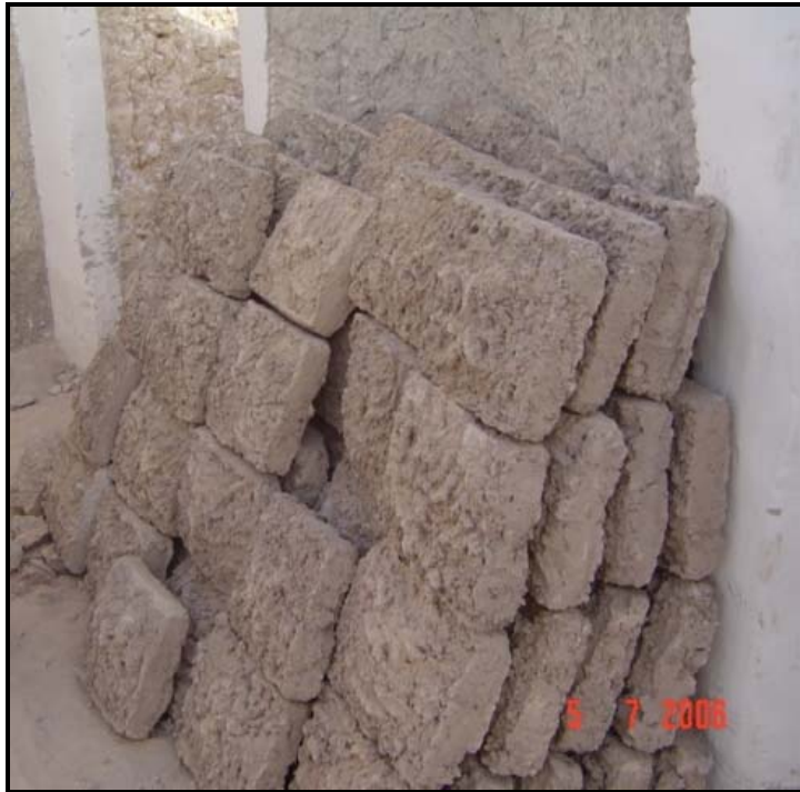
Figure 4.42 Local mud brick of Ghadames.
