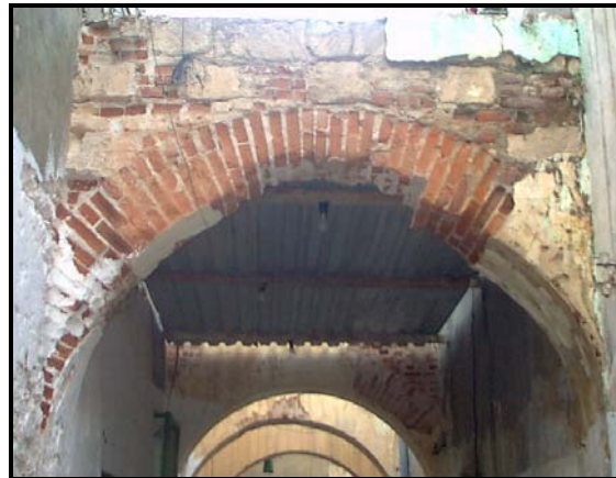
Figure 2.22 Use of brick in arch construction. (Source: Bash-Imam and Bukra, 2004. )
