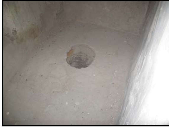
Figure 4.47 Toilet room of the traditional house in Ghadames.
