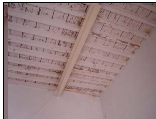
Figure 4.14 Timber ceiling in the traditional house in Tripoli.
