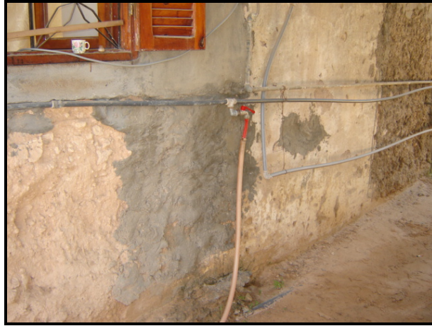
Figure 4.17 Water supply pipes added later to the traditional house in Tripoli.
