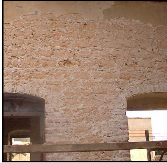
Figure 2.21 A wall constructed from limestone. (Source: Bash-Imam and Bukra, 2004. )
