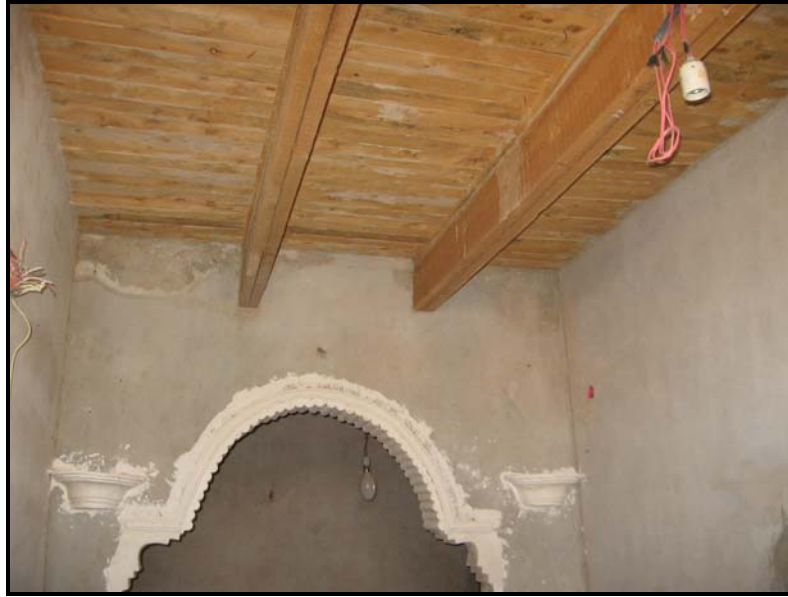
Figure 4.7 Wooden ceiling of a house in Tunes.
