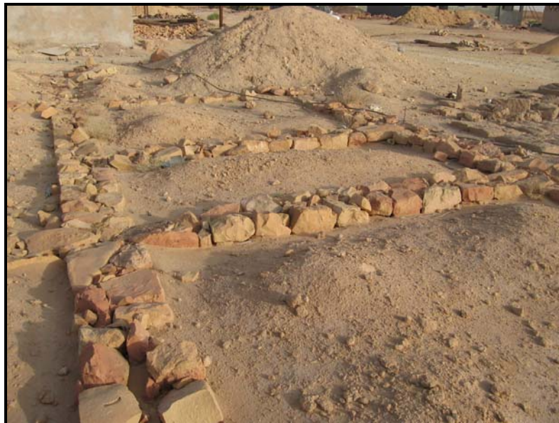
Figure 4.6 Volcanic stone foundations of a house in Tuneen.
