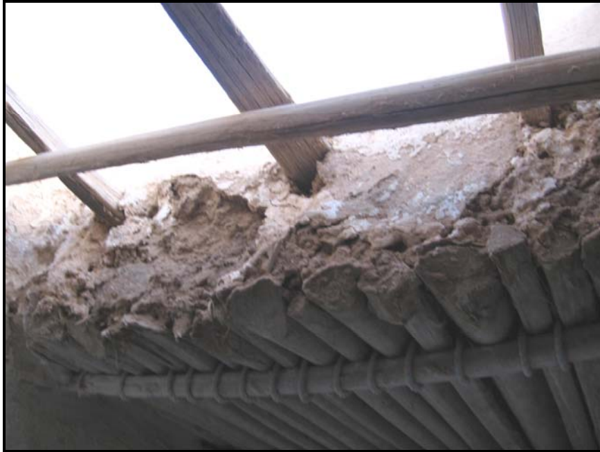
Figure 4.45 Mud mortar and timber ceiling of the traditional house in Ghadames.
