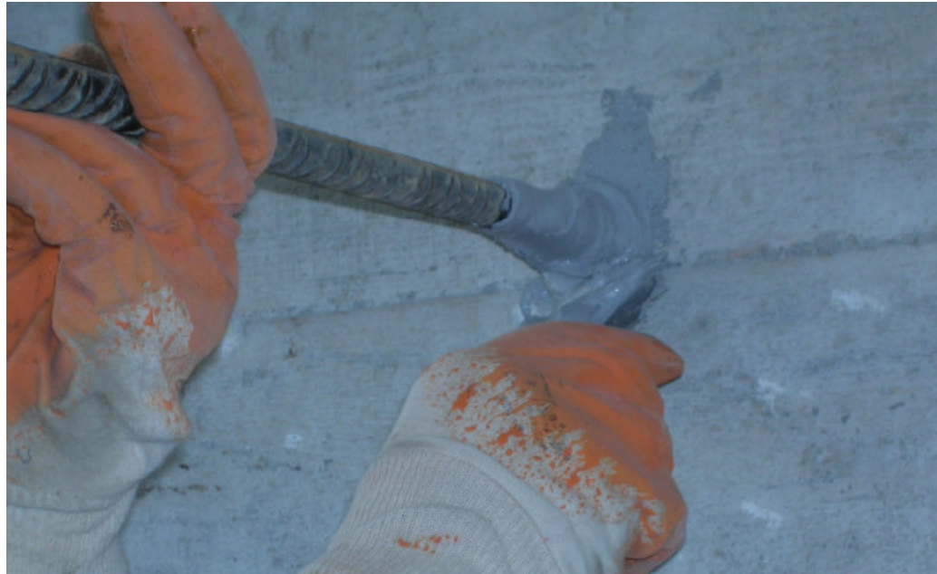
Figure 3.8 Placing of the anchors
