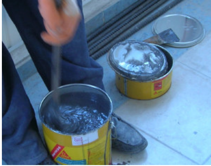
Figure 3.7 Mixing the two components of the adhesive
