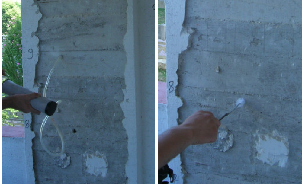
Figure 3.6 Cleaning of the holes
