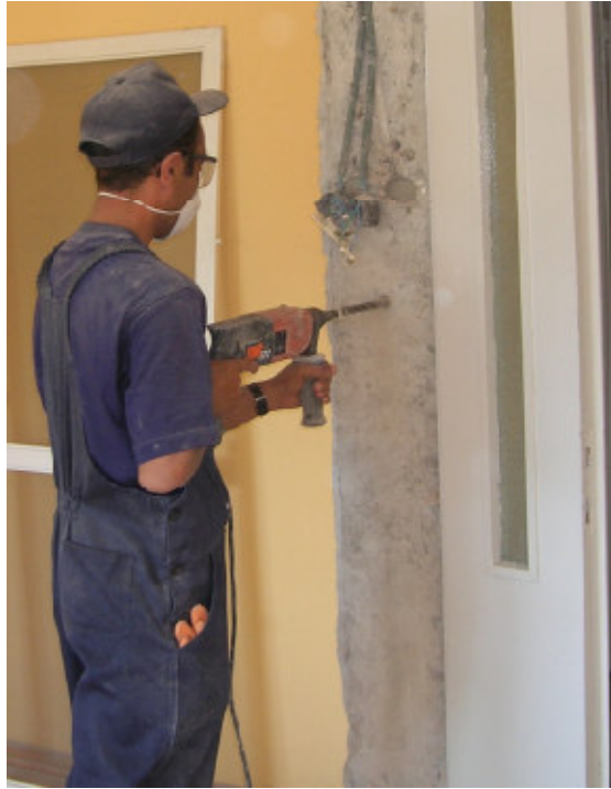
Figure 3.5 Drilling of the holes
