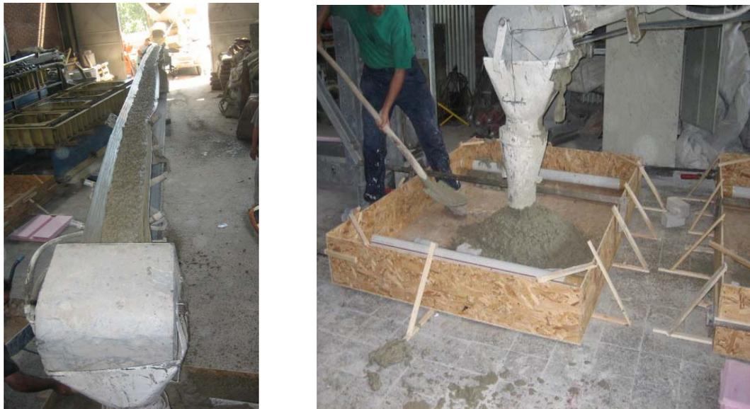
Figure 3.1 Concrete being placed in the laboratory
