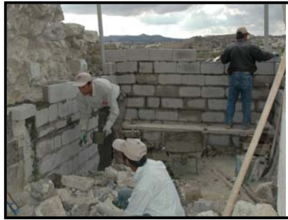
2.43 Construction of brick walls
