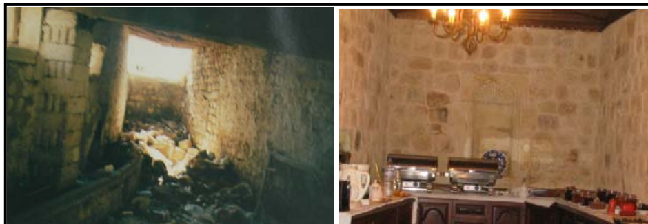
Figure 2.91 Partially collapsed south wall was reconstructed
