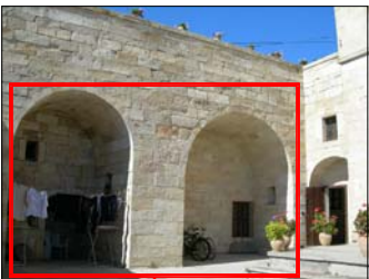
ARCHES WERE RECONSTRUCTED BY REUSED STONES. THEIR DIMENSIONS WERE CHANGED. BECAUSE OF USING REUSED STONES IT IS NOT UNDERSTOOD THAT WALLS ARE ALTERATION.
