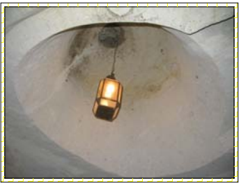
DIRECT ILLUMINATION WAS PROVIDED BY LIGHTING ELEMENTS HANGING INSIDE THE CHIMNEYS
