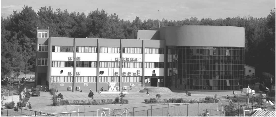
Figure 3.1. View of Case Study 1 building on completion.
