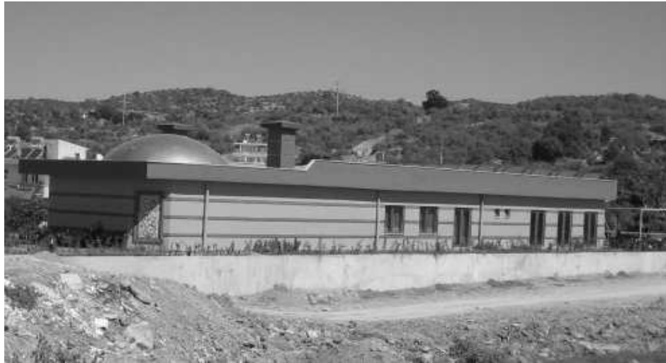
Figure 3.10. View of Case Study 6 building on completion.
