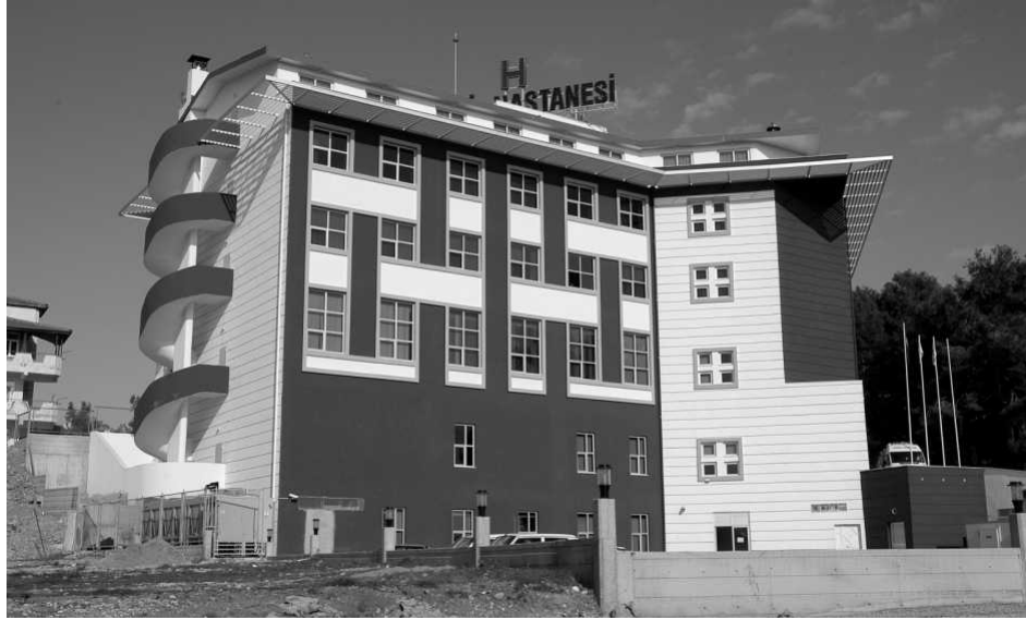
Figure 3.2.b. View of Case Study 2 building on completion.
