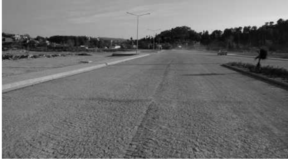
Figure 3.6.a. View of Case Study 4 on completion.
