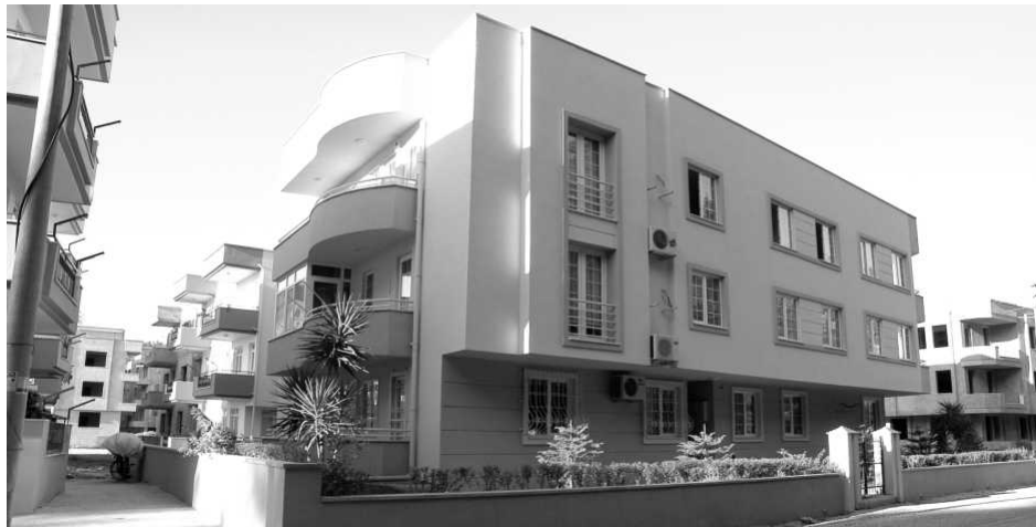
Figure 3.4.b. View of Case Study 3 building on completion.
