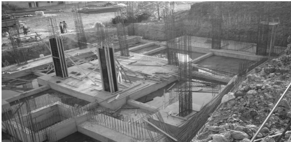
Figure 3.2.a. View of Case Study 2 building during construction.
