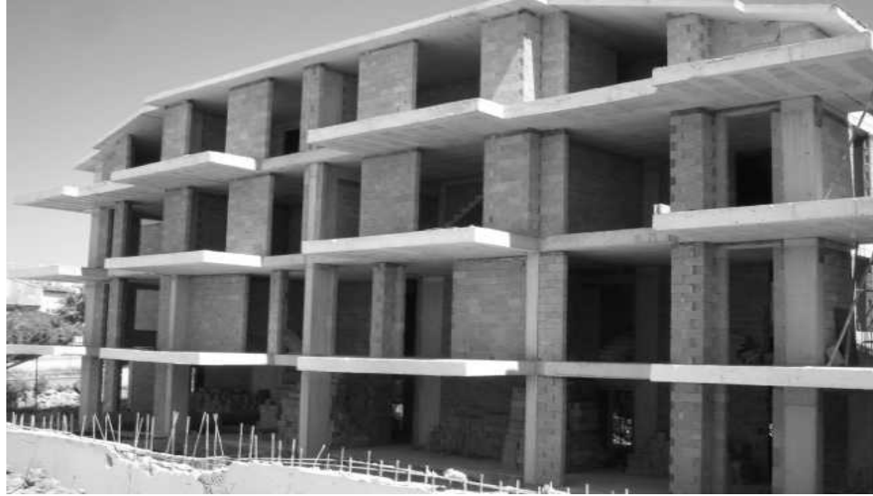
Figure 3.13.a. View of Case Study 8 building during construction.
