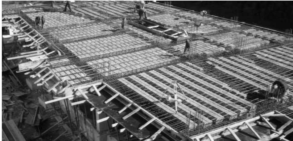
Figure 3.4.a. View of Case Study 3 building during construction.
