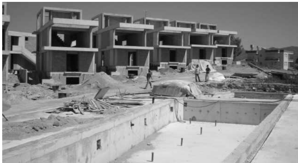
Figure 3.8.a. View of Case Study 5 buildings during construction.
