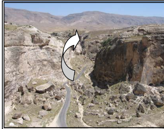
Figure 2.6 The location of the main canal, the siphon and the Pool
