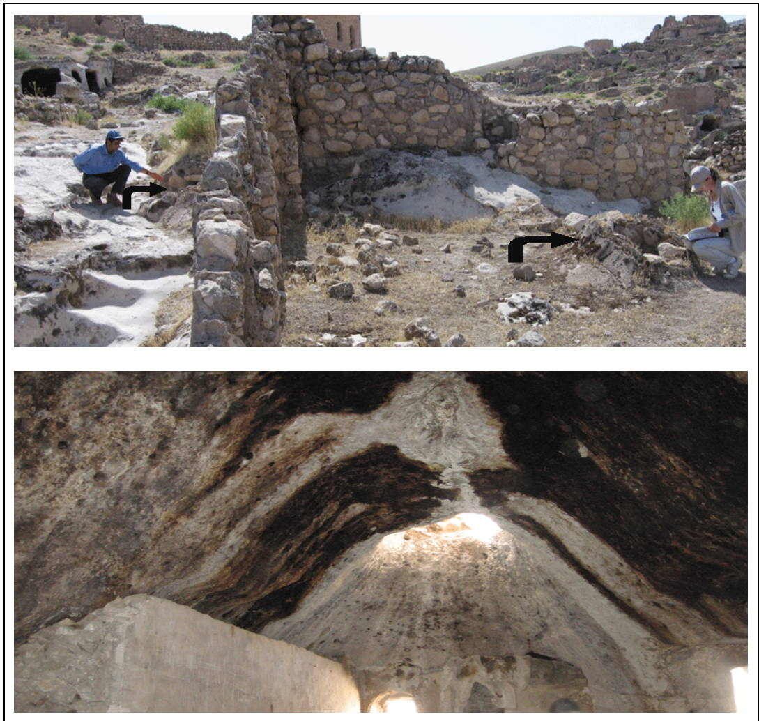
Figure 3.18 Sample for two-chimney cistern. External view (top) shows the location of the chimneys (black arrows). The lower view shows the interior part of the cistern.
