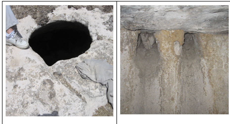
Figure 3.41 Canal extensions observed from the interior facade of B39 unit
