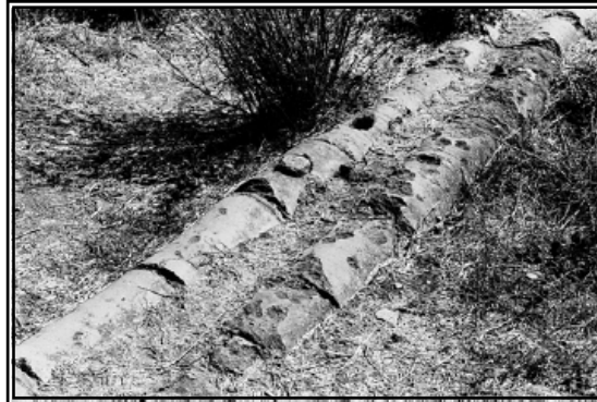
Figure 6.3 Pipeline segments with top air holes in Ephesus
