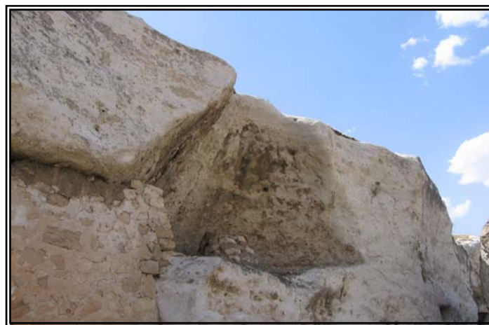
Figure 5.3 A destroyed cistern whose half is absent in D26
