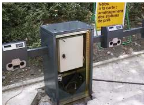
Figure 4.13 Station controller ( http://www.creacom.be/Smartbike/index.htm )
