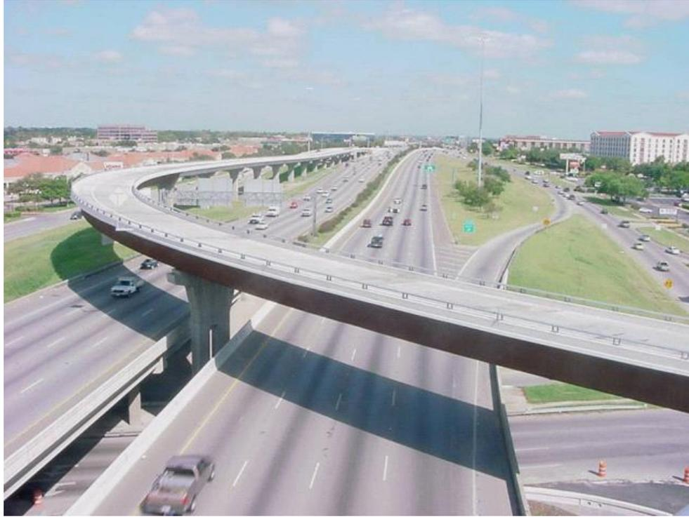
**Fig.1.3. A Photo of a Curved Box Composite Bridge**
