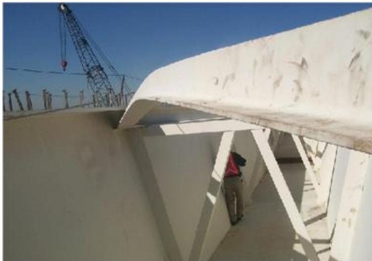
**Fig.1.4. Buckling of a Brace Member in a Curved Box Girder Bridge**
