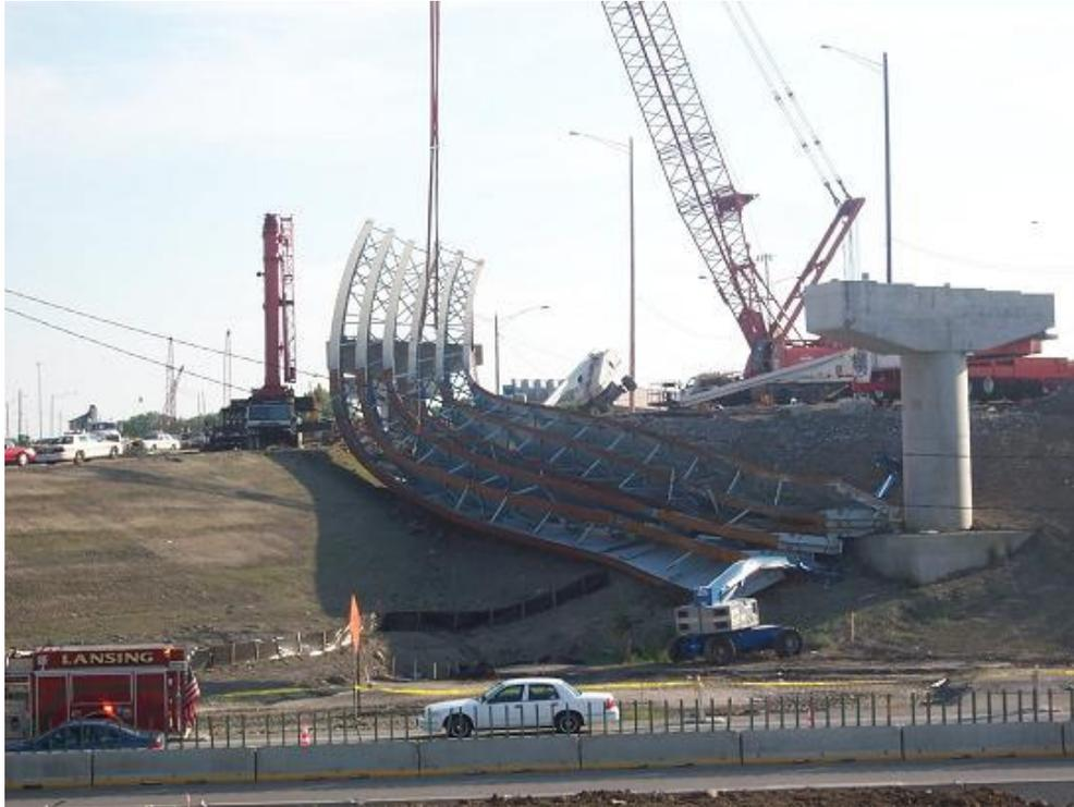
**Fig.1.5. Complete Collapse of a Curved I-girder Bridge**
