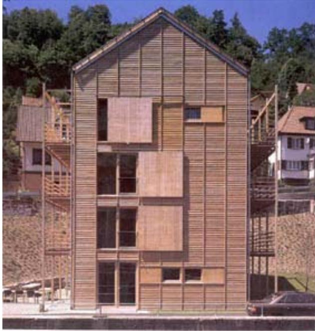
**Figure 6.2. River facade with external sliding shutters.**
