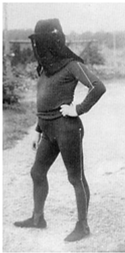
Figure 2.1 Marey's motion capture suit
