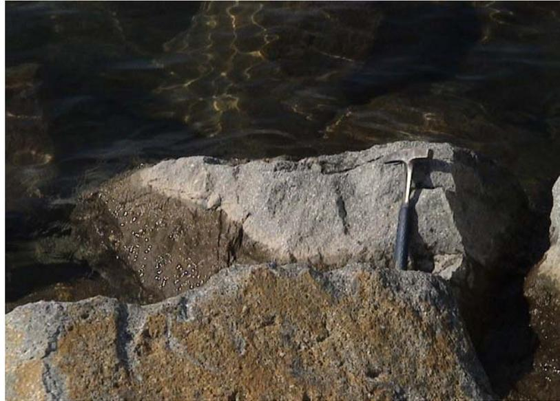
Figure 6.3 A close up view of the Çömlekçikuyu andesite in the Hisarönü breakwater
