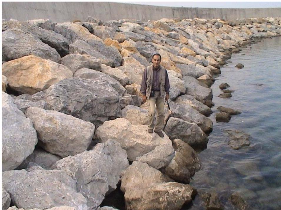
Figure 6.7 A close up view of the Tarlaağzı limestone used in the Tarlaağzı breakwater
