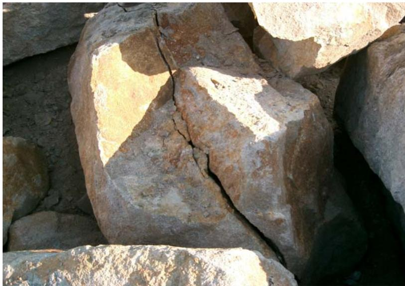
Figure 6.4 Andesite blocks containing cooling joints in Hisarönü breakwater
