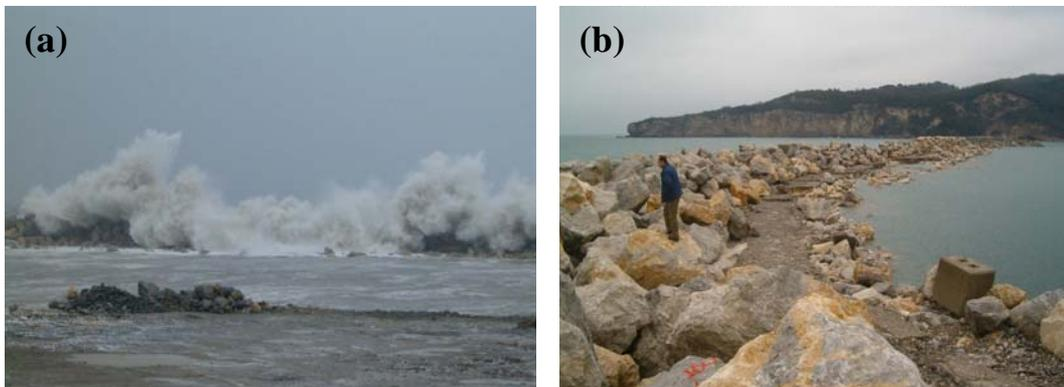
Figure 1.1 A destructive five meter high wave impacting the Tarlaağzı ship shelter as a result of the February 2004 storm (a) and the resulting damage at the shelter (b)
