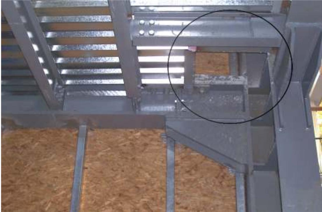
**Figure 4.36.** A view showing the hole on the steel deck for the installation channel
