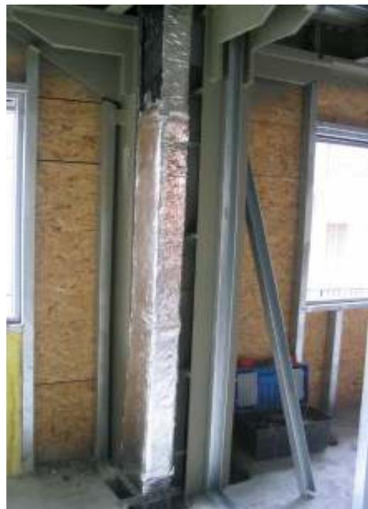
**Figure 4.35.** A view showing the conduit installed next to the column
