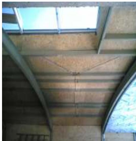
**Figure 4.8.** Curved steel beams
