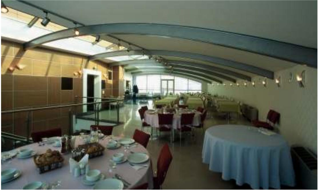
**Figure 4.37.** Curved beams supporting the roof
