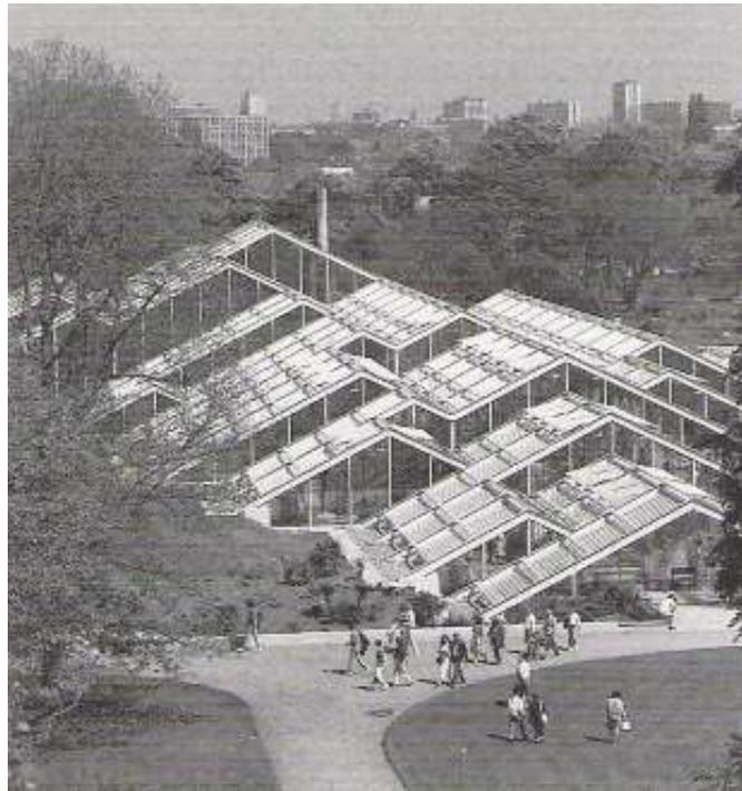
**Figure 2.28.** Pitched roof structure: Princess of Wales Conservatory in London, England (Source: Plank, 1993)
