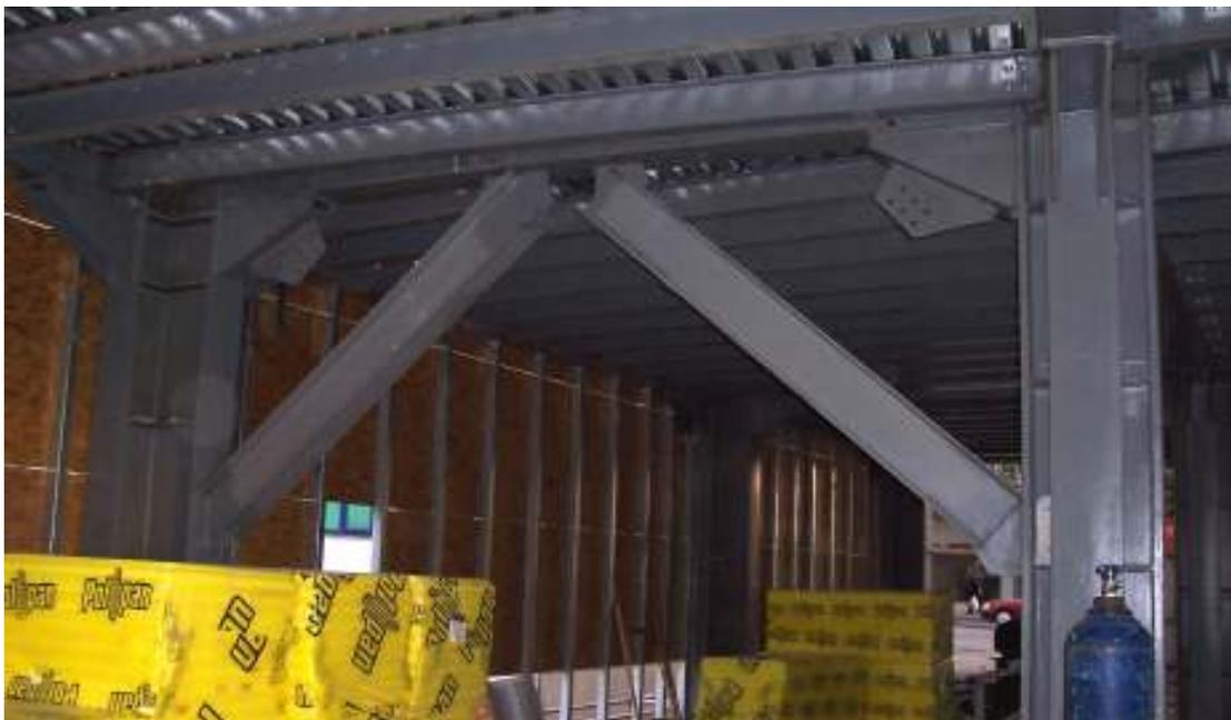
**Figure 4.32.** Rectified structural bracing
