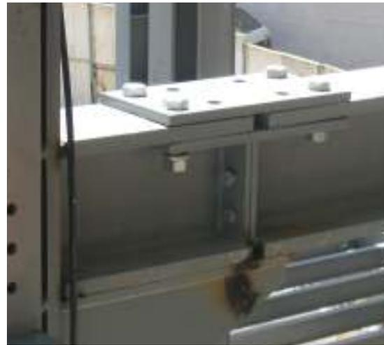
**Figure 4.13.** Column-beam connection with splice (fish) plates
