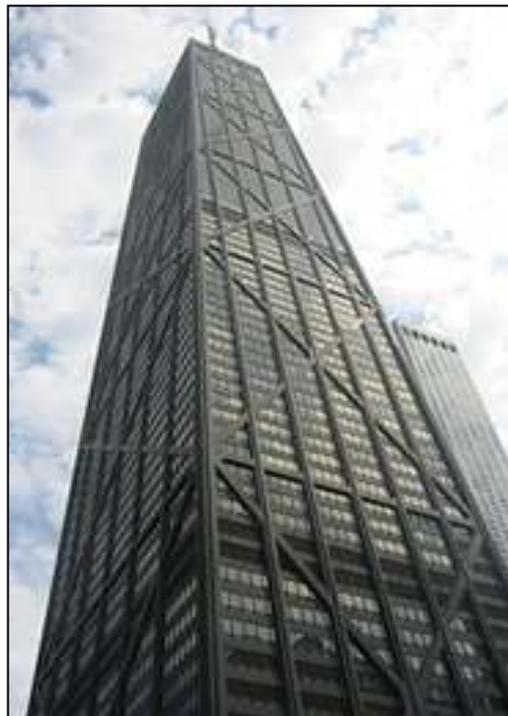
**Figure 2.12.** Use of external steel bracings in the John Hancock Center in Chicago, USA (Source: [www.hispago.com](http://www.hispago.com), retrieved 2006)
