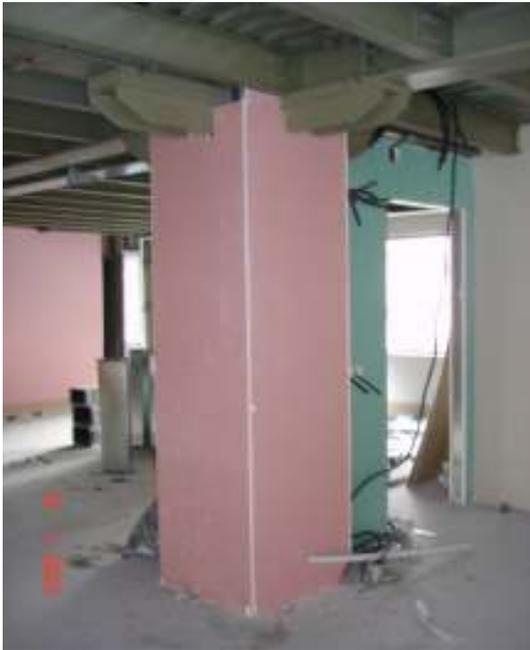
**Figure 4.24.** The steel column and the installation channel enclosed within gypsum board casing
