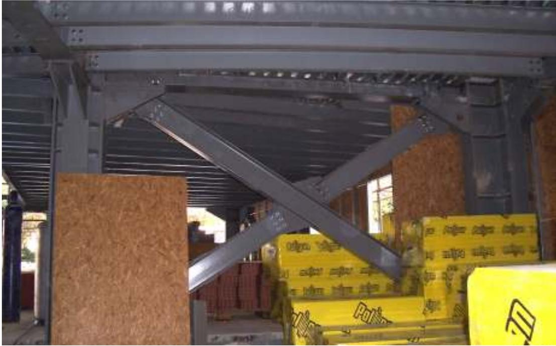
**Figure 4.31.** Incorrect structural bracing
