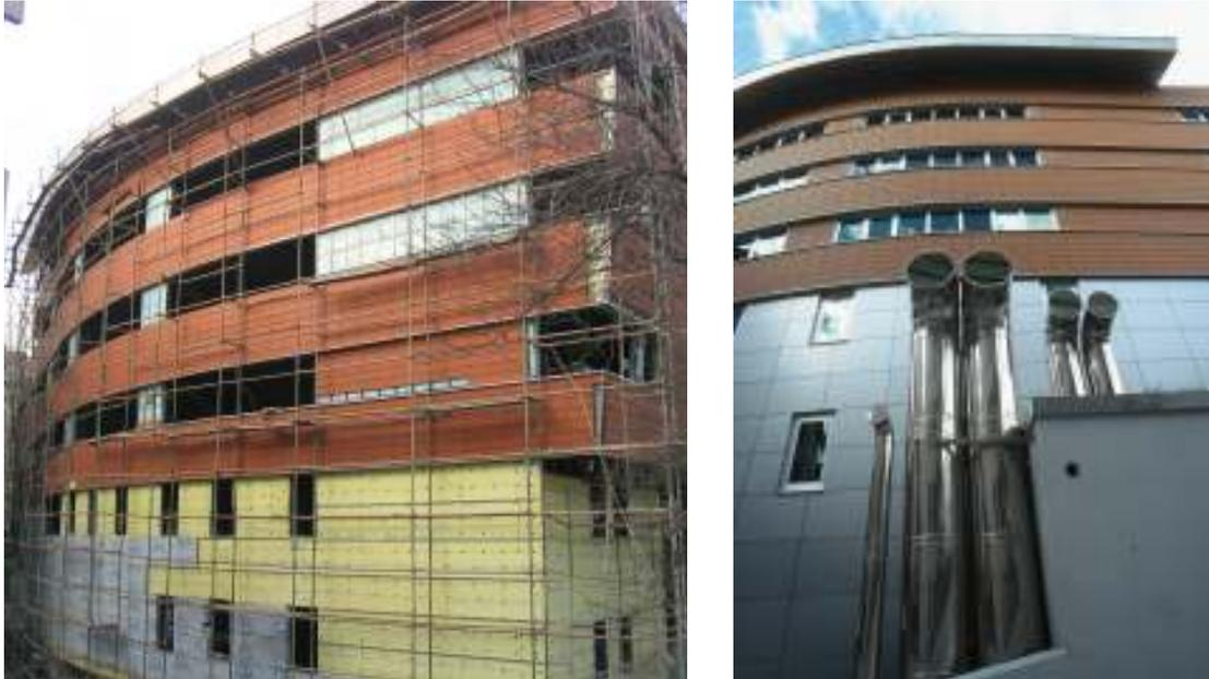
**Figure 4.22.** Construction of the curtain wall and its final photo
