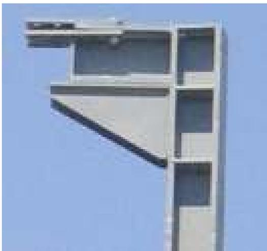
**Figure 4.12.** A free-standing column before connecting the beams
