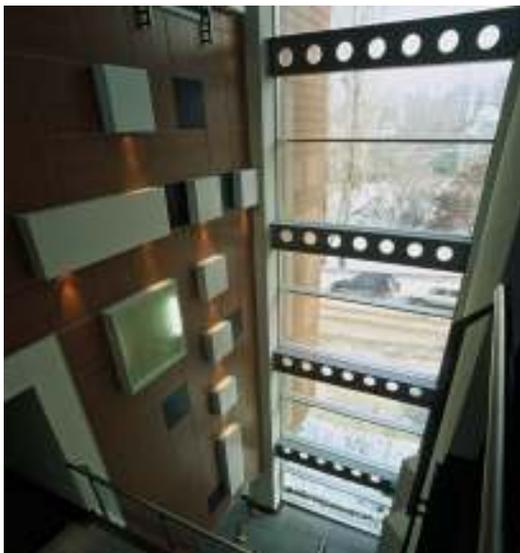
**Figure 4.7.** Perforated steel beams
