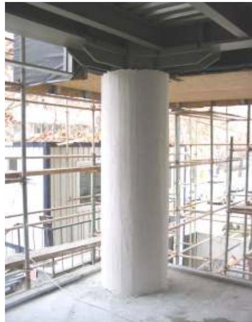
**Figure 4.25.** Circular encasement for columns at the façade
