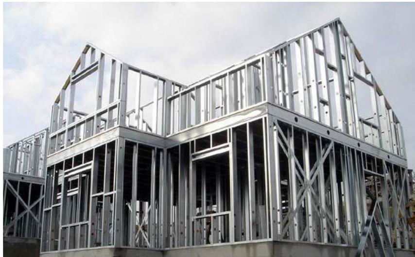
**Figure 2.45.** A view of the steel-framed house in Istanbul, Turkey, during its construction phase (Source: [www.zeytinsuyutepesi.com](http://www.zeytinsuyutepesi.com), retrieved 2006)
