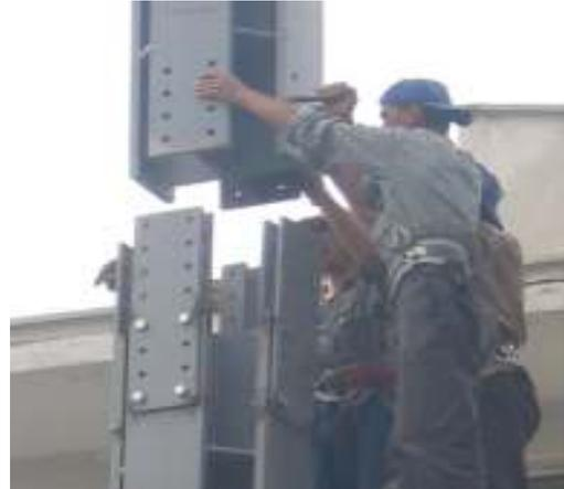
**Figure 4.17.** Assembly of the columns by using splice plates
