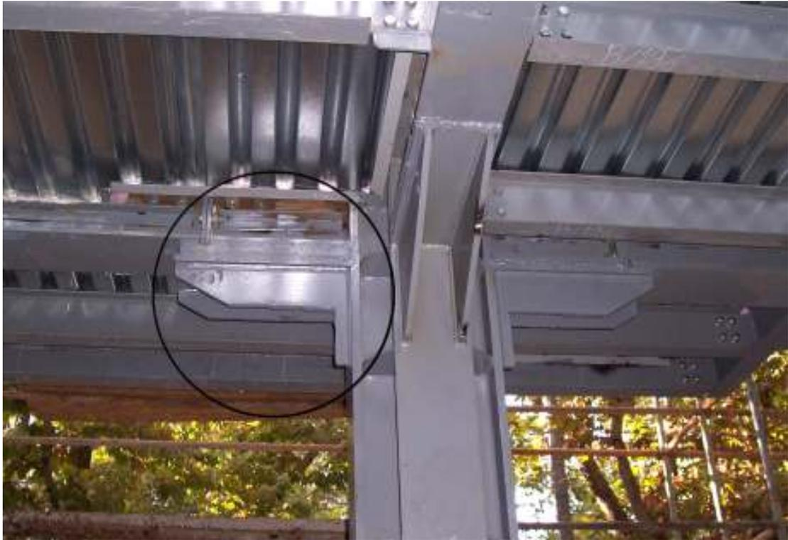
**Figure 4.33.** The modification made on gussets
