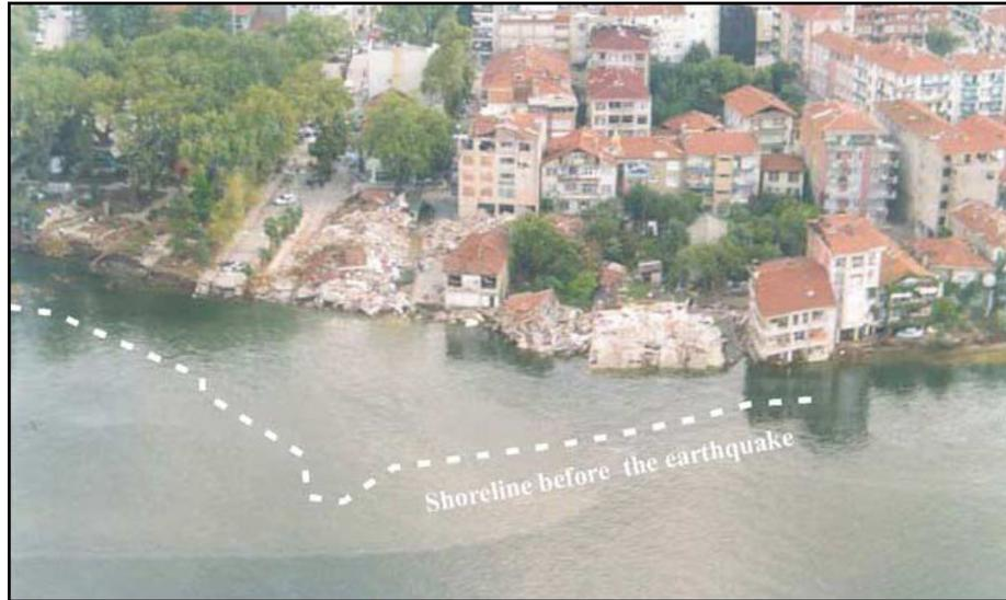
Figure 3.9 Çınarlık shore after earthquake (Çetin et.al, 2004.a)
