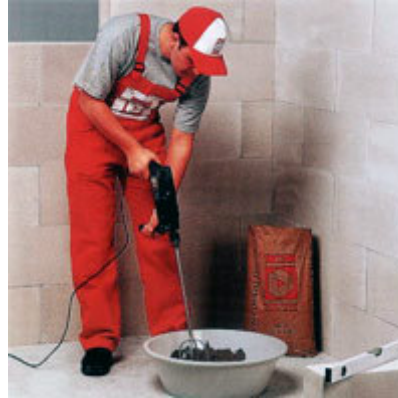
Figure 2.12. Preparation of the adhesive mortar ( www.akg-gazbeton.com )
