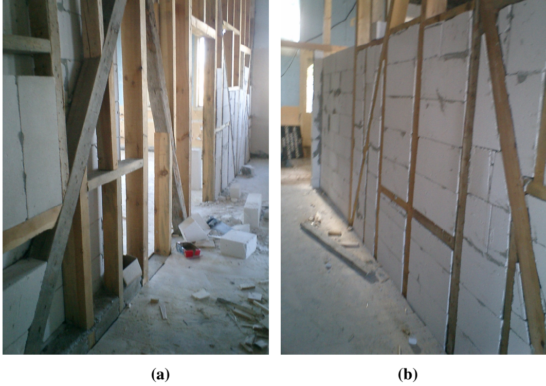
Figure 2.18. Öğretmen Evi, Safranbolu (a) close view to the application of AAC inside the timber framed structure (b) the timber framed wall with AAC infill after the repair work
