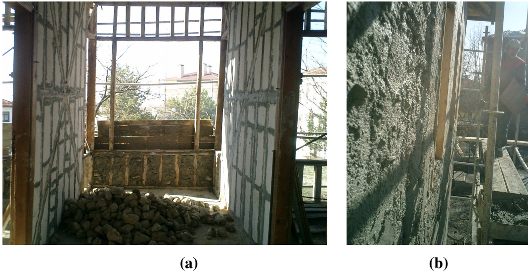
Figure 2.16. The Kindergarten in Safranbolu, (a) a view showing the use of AAC as an infill material substitute of the original stone infill (b) a view from the outside showing the application of the exterior cement based plasters over the timber framed structure with AAC infill.
