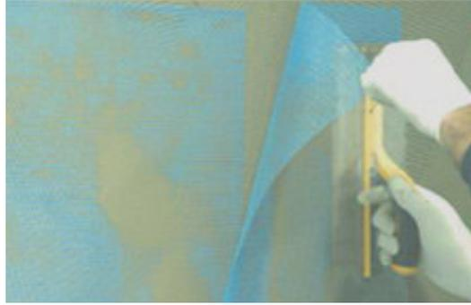
Figure 2.3. Application of thermal insulation undercoats with reinforcing mesh
