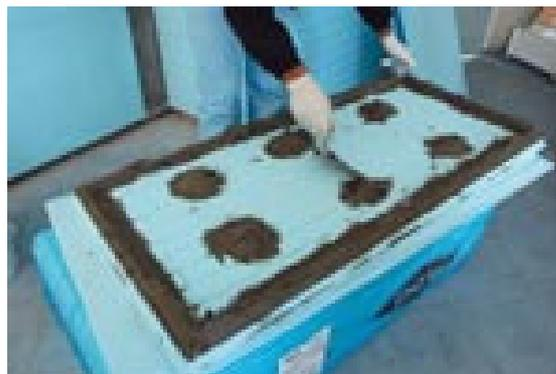
Figure 2.2.b. Application of bedding plaster to thermal insulation board by ribbon and dab method (www.bulak.net, 2006)
