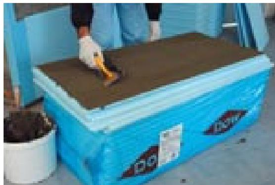
Figure 2.2.a. Application of bedding plaster to thermal insulation board by notched trowel method (www.bulak.net, 2006)
