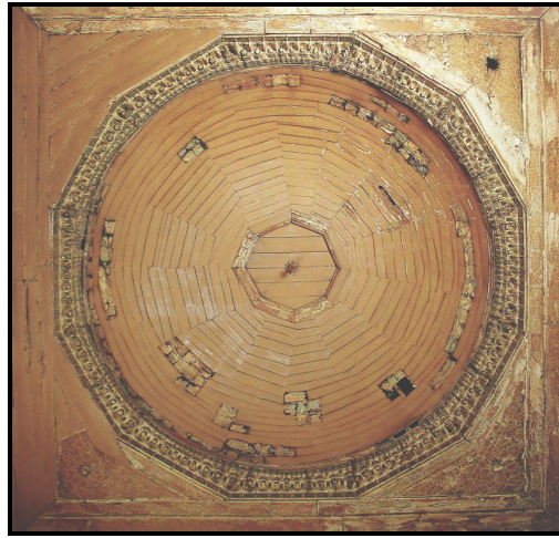
Figure 73: Wooden dome of the main hall of hünkar kasrı , Yeni Valide Complex courtesy of Hatice Karakaya
