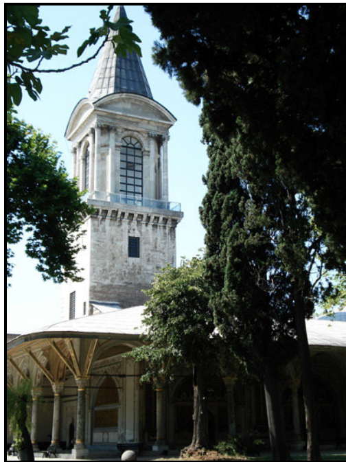
Figure 15: Tower of Justice and the Court Hall below, photographed by the author
