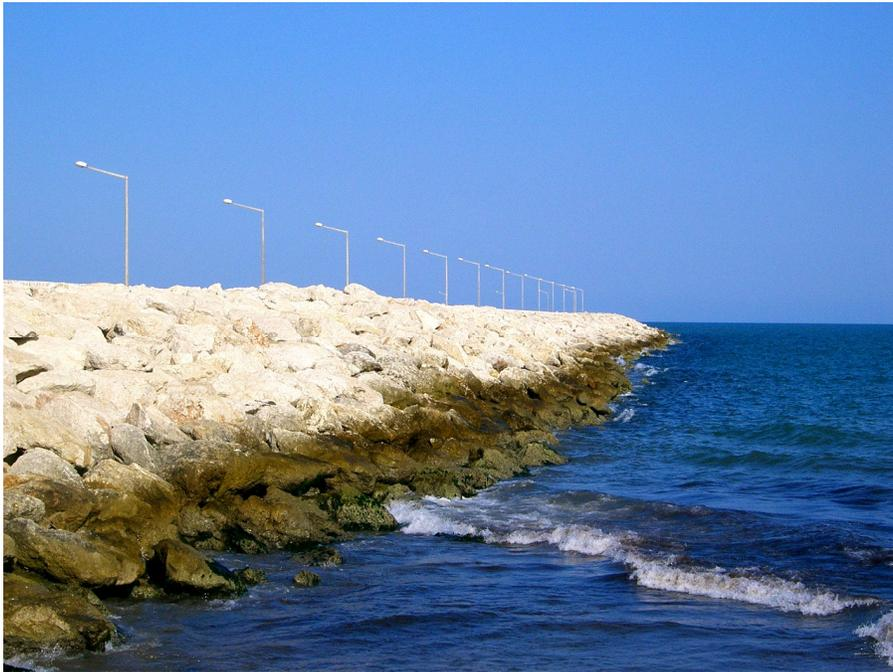
Figure 6.2 Limestone blocks used in the Mersin harbour with wetting-drying effects after 1 year.
