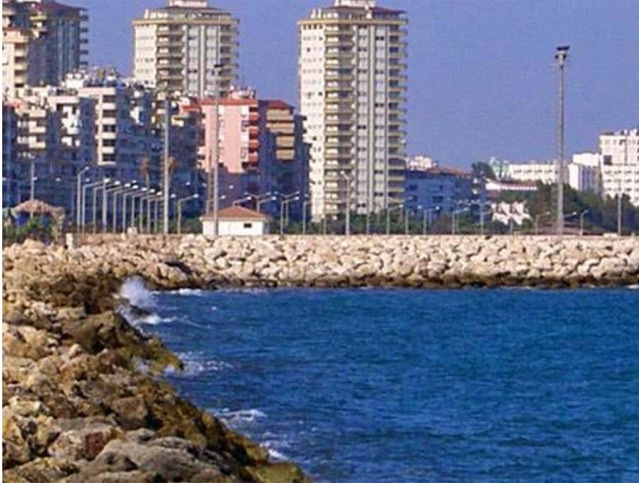
Figure 1.1 A view of armourstones used in Mersin harbor.
