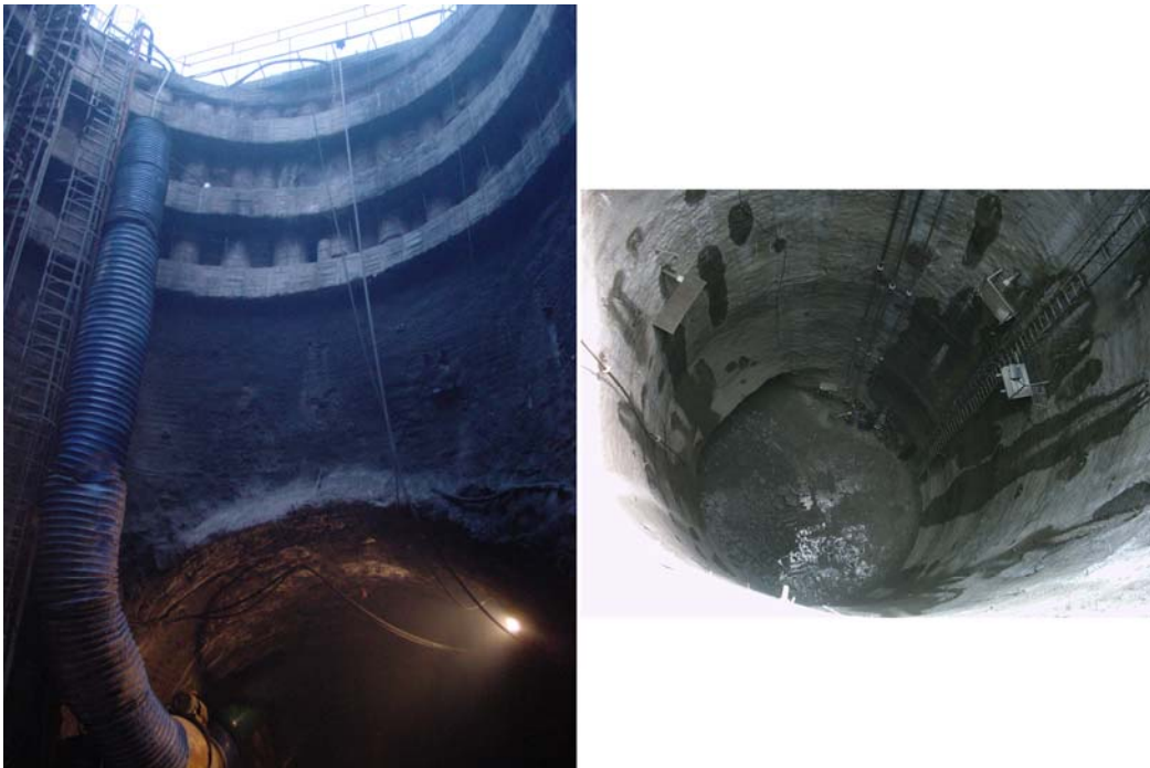
Figure 2.4 A view of the shaft access
