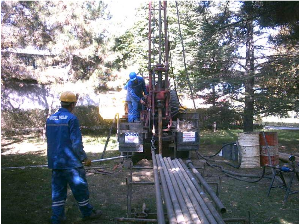
Figure 2.14 Photo image showing borehole drill
