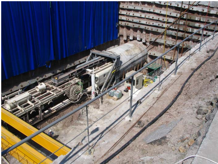
Figure 2.26 TBM and segment installation
