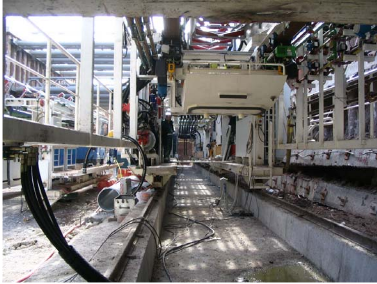
Figure 2.25 Assemblage of TBM at Dışkapı station
