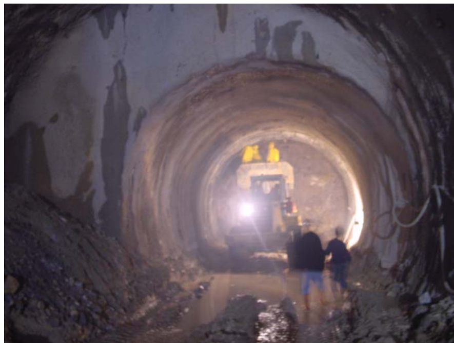
Figure 2.10 A view from the platform tunnel cross-section
