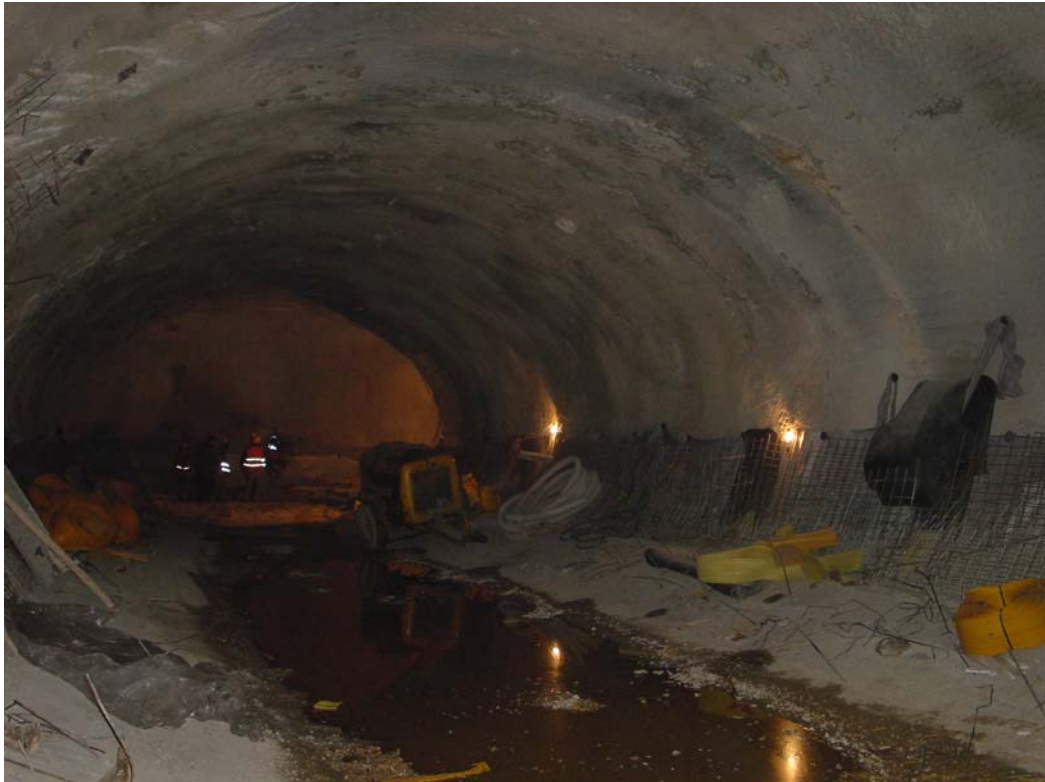
Figure 2.12 Photo image showing connection tunnel
