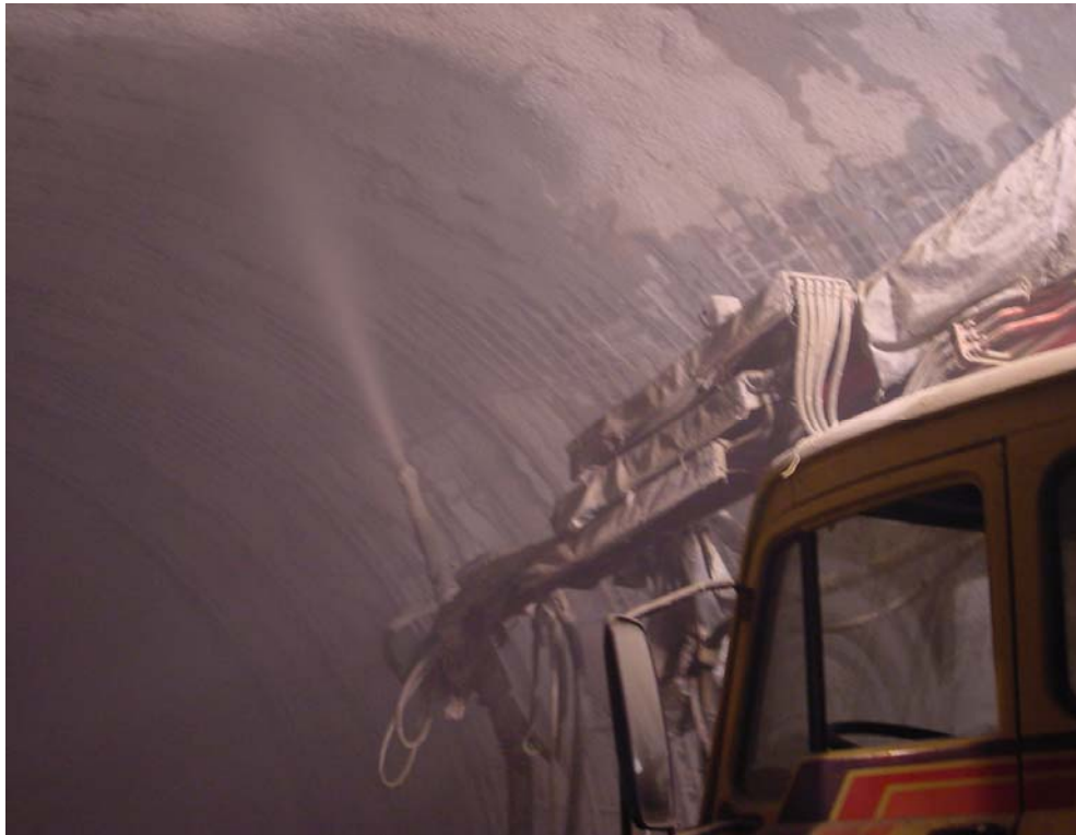
Figure 2.1 Photo image showing shotcrete application
