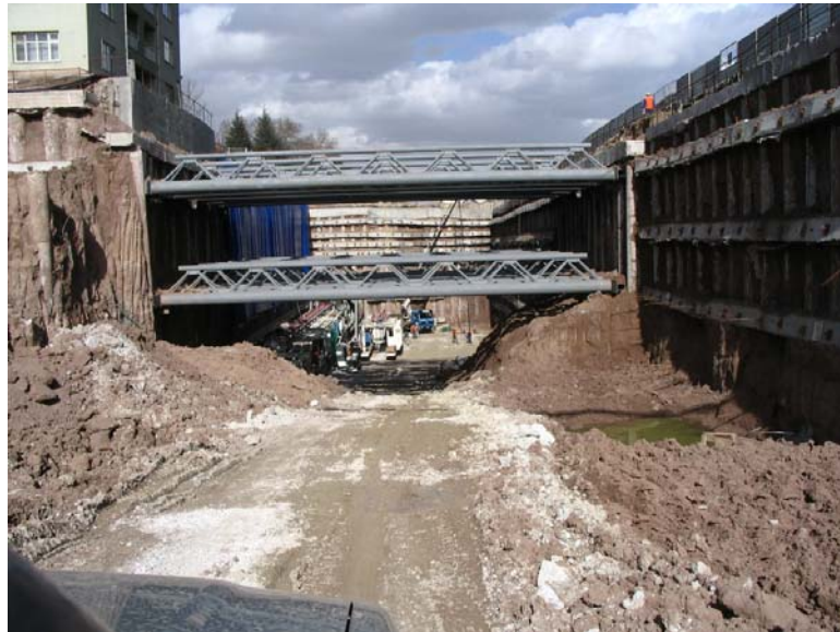
Figure 2.24 Open excavation for tunnel portal approach at Dışkapi.
