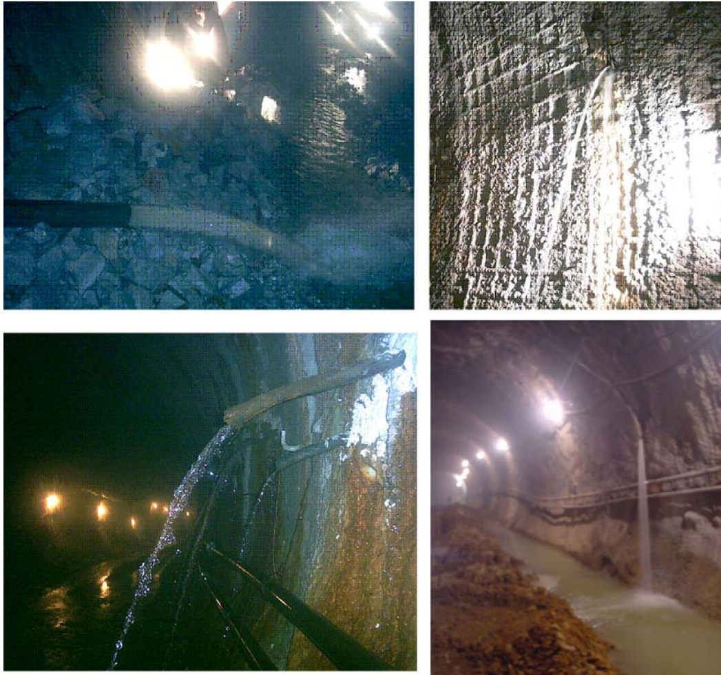
Figure 2.23 Groundwater inflow to the tunnel
