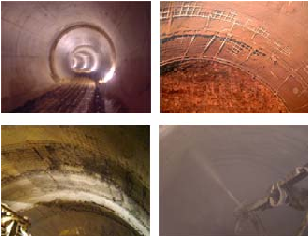
Figure 2.3 Support measures: steel ribs, shotcrete, wire mesh, and concrete lining
