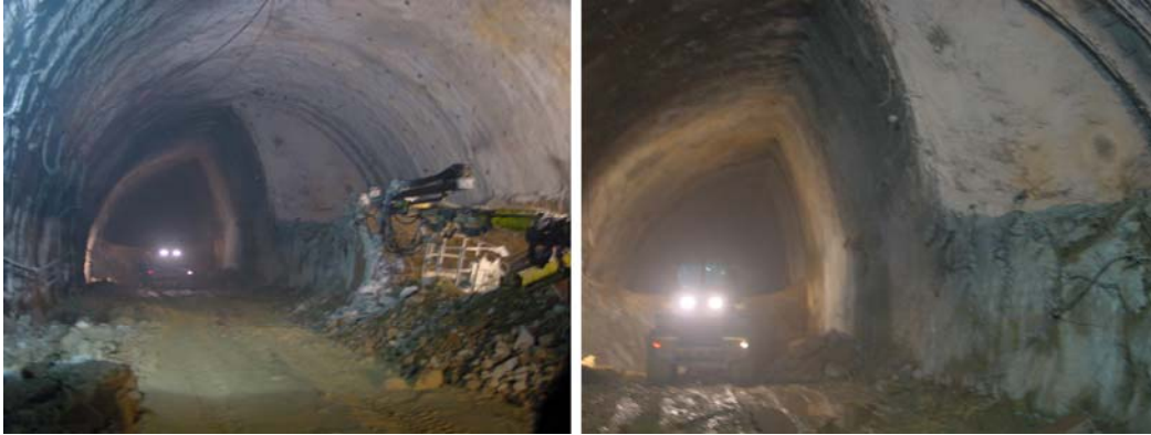
Figure 2.8 Photo images illustrating six phase excavation: close and far
