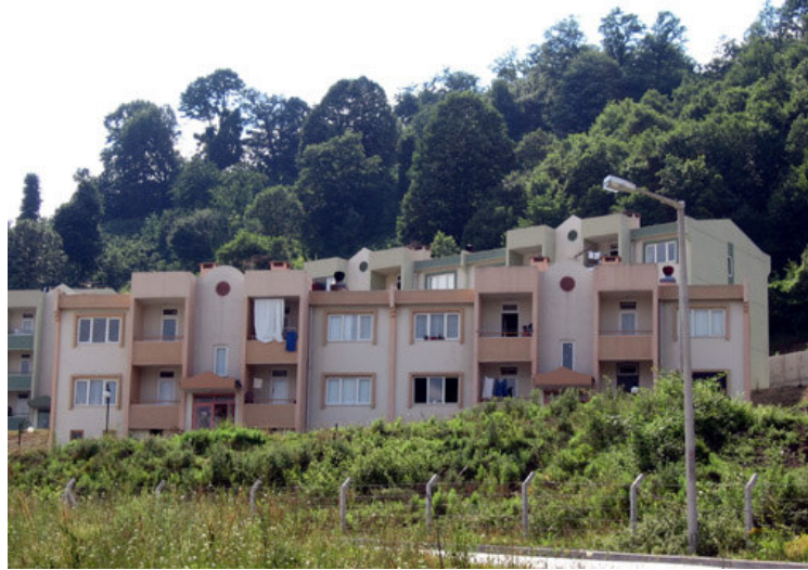
Figure V.2: Permanent Houses built by the government. Gölyaka, Düzce.
