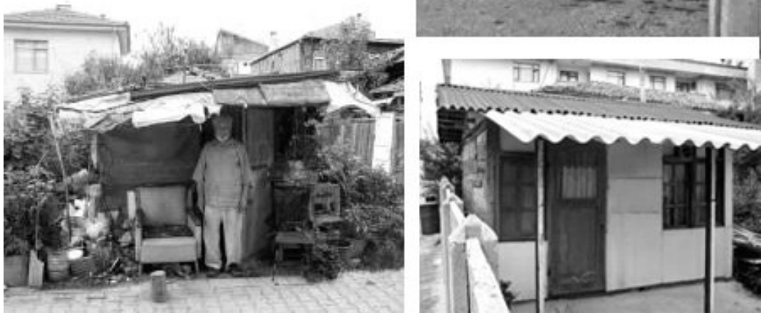
Figure II.3: Examples of sheltering built after the August 17 th earthquake. Adapazarı, 2001.
