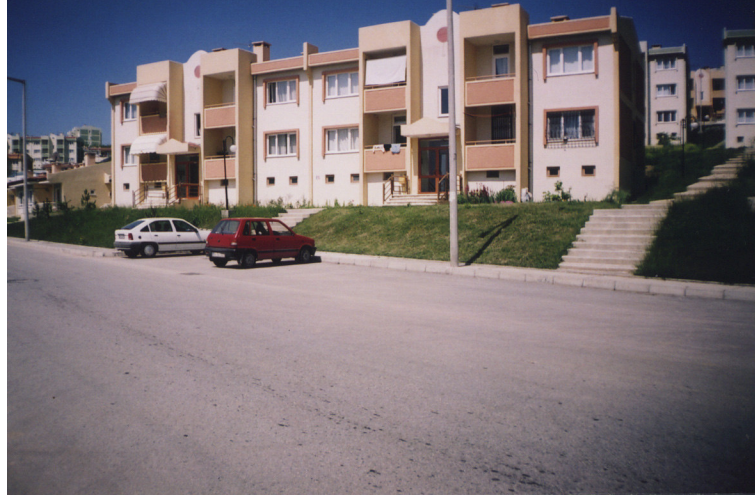
Figure V.1: Permanent Houses built by the government. Camili, Adapazarı.
