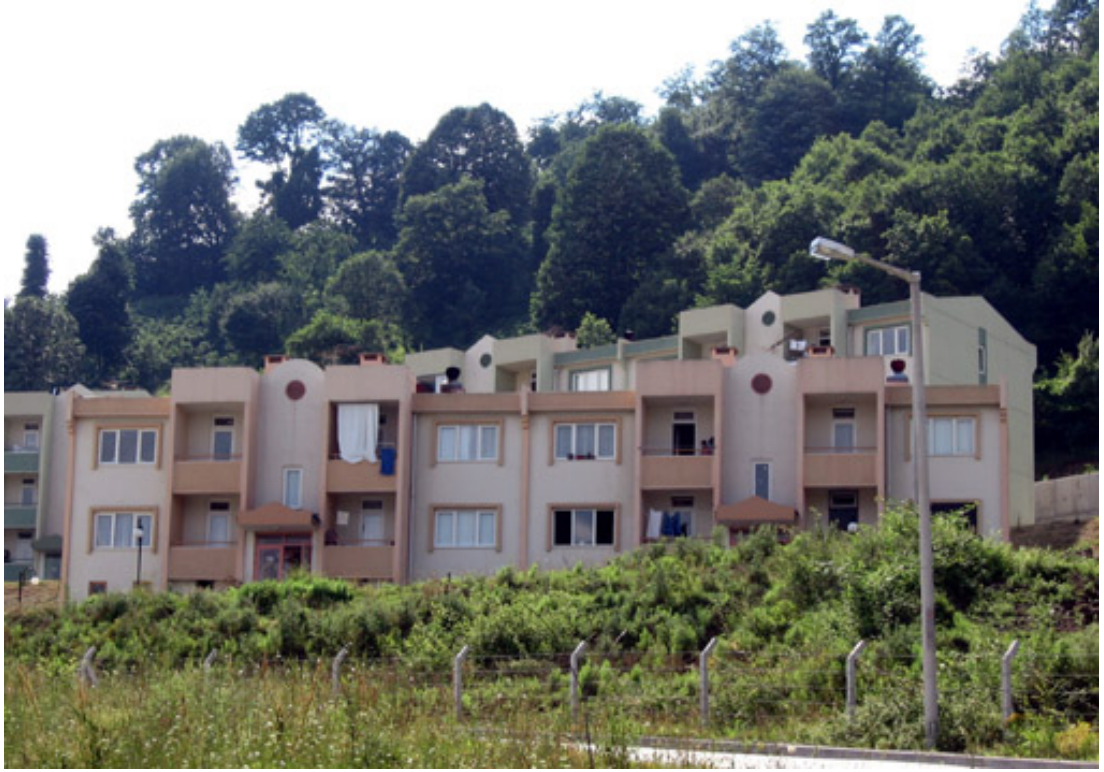
Figure III.3: Site view of the Gölyaka Permanent Houses. Gölyaka, 2005.
