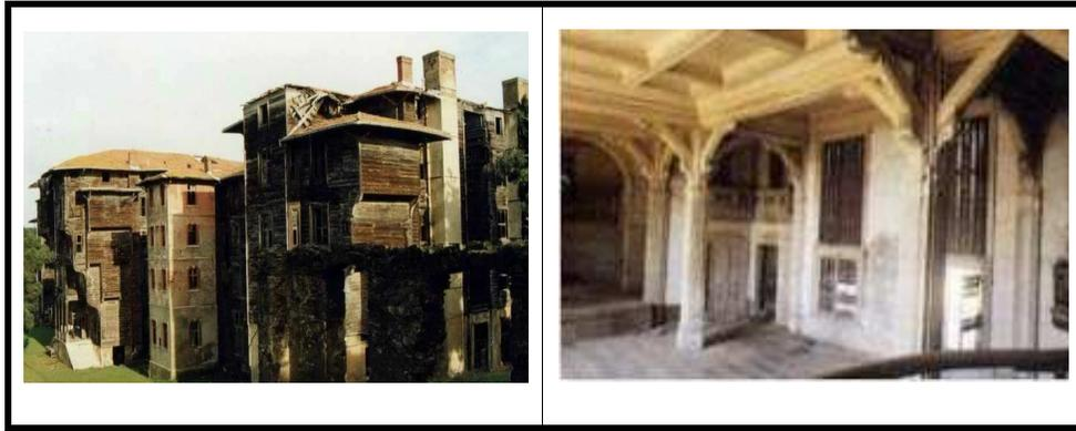
**Figure III. 38** Büyükada Rum Orphanage<sup>26</sup> is a building that have a totally timber structure (Adalar Governership, document on-line).
