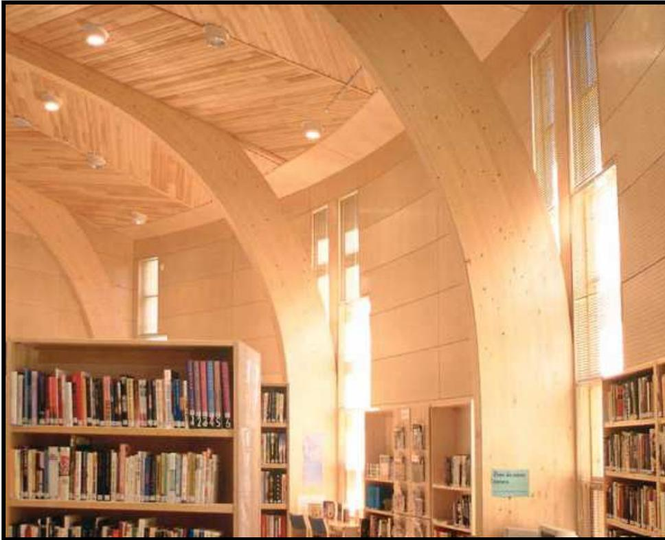
**Figure II. 56** Roof structure of the Eno Library; Eno, Eastern Finland (Timber Research and Development Association, document on-line).
