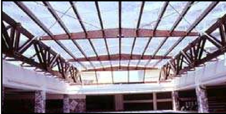
**Figure III. 36** Roof structure for the indoor swimming pool of Lares Hotel<sup>24</sup> with timber trusses (Oran Mimarlık, document on-line).
