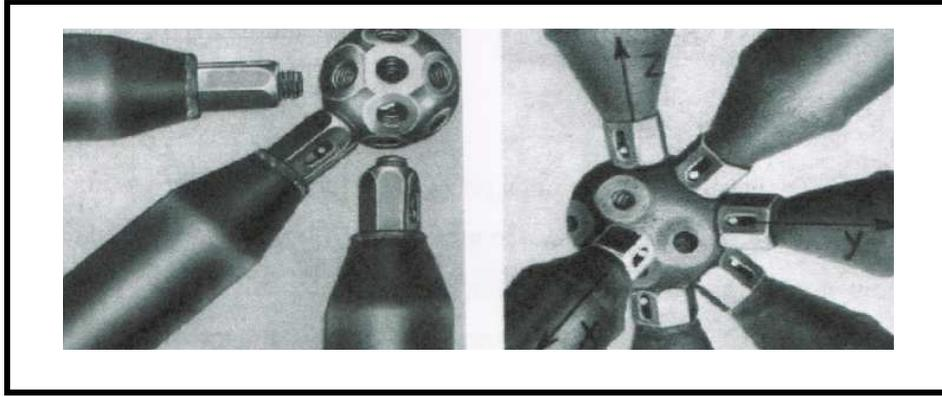
**Figure II. 47** Node points in a space frame (Orbay and Savaşır, 2004:41).
