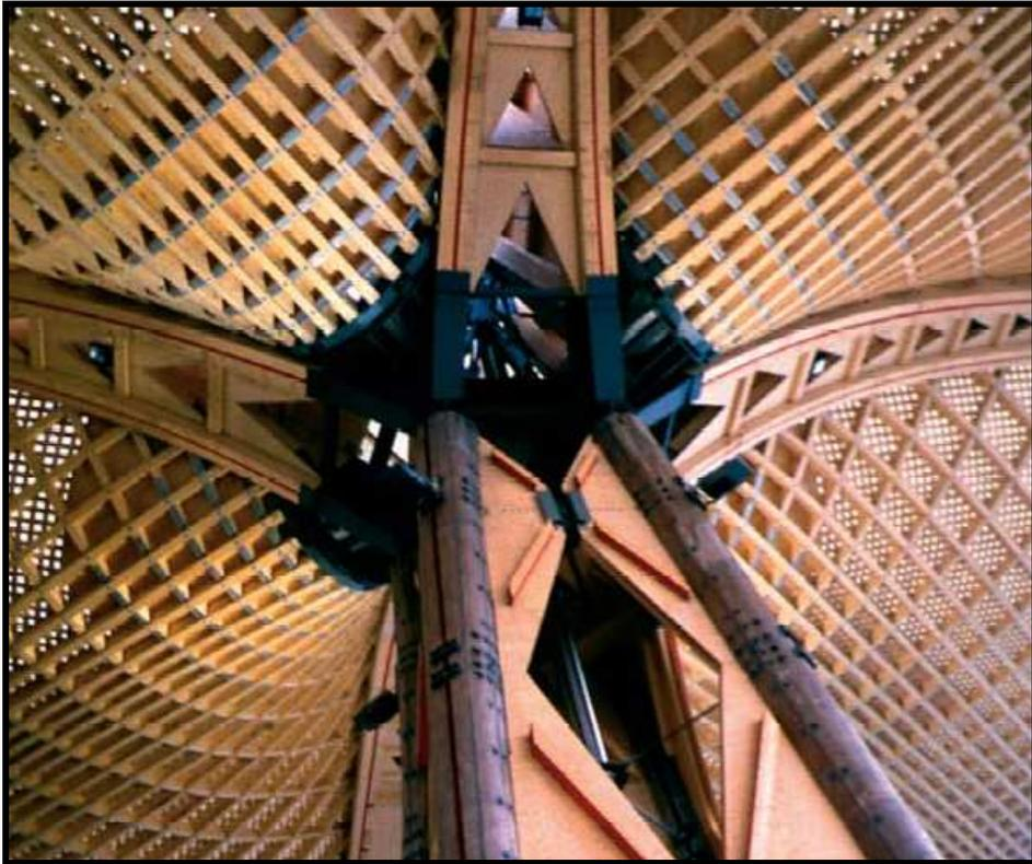
**Figure II. 53** Roof structure of the Hanover Expo Canopy<sup>10</sup>; Hanover, Germany (Timber Research and Development Association, document on-line).
