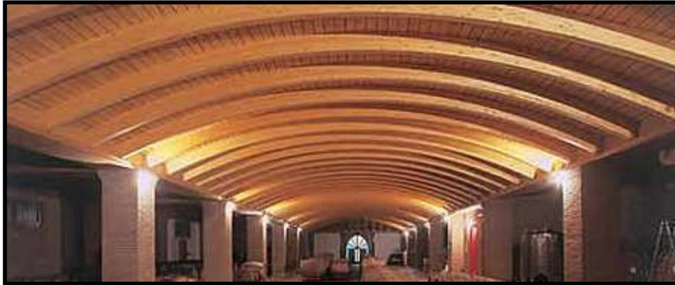
**Figure II. 32** Arch structure of Cantina Fossoli; Colognola, Italy; Architect: Antonio Masconi (Holzbau Spa, document on-line).
