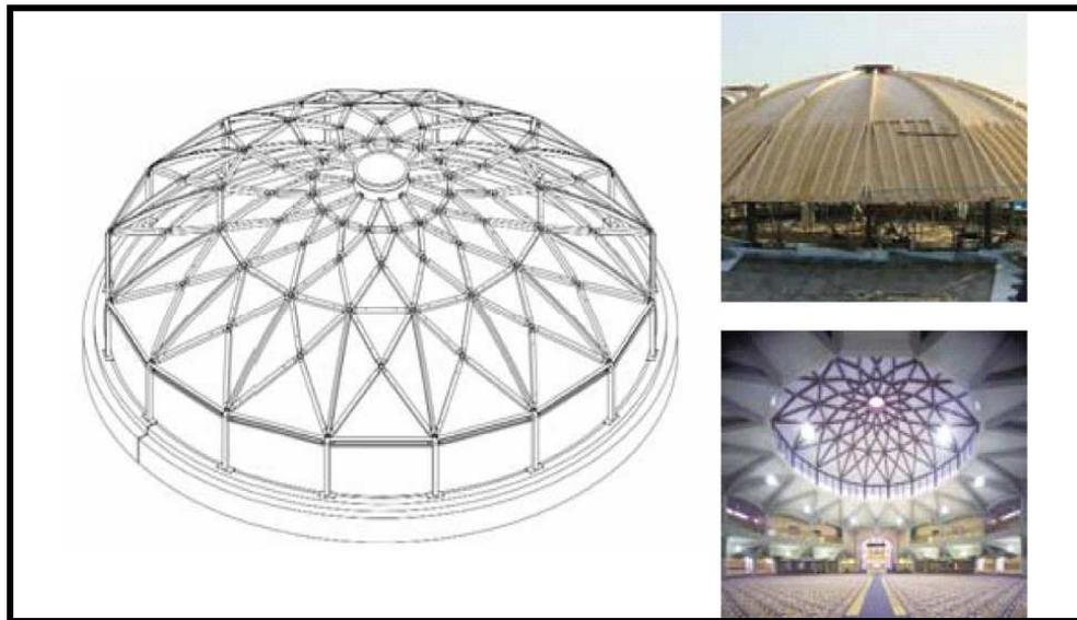
**Figure II. 61** Roof structure of the Gurdwara Southall Temple<sup>12</sup>; London (Timber Research and Development Association, document on-line).
