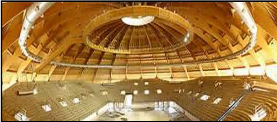
**Figure II. 64** Roof structure of Livorno Palasport<sup>13</sup>; Livorno, Italy (Holzbau Spa, document on-line).
