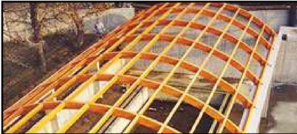
**Figure III. 37** Roof structure for the indoor swimming pool of Aytek indoor swimming pool<sup>25</sup> with timber vaults (Oran Mimarlık, document on-line).
