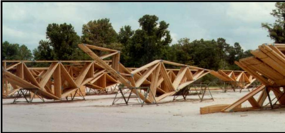
**Figure III. 12** Manufactured trusses are stored on site in a proper manner (MiTek Solutions, document on-line).
