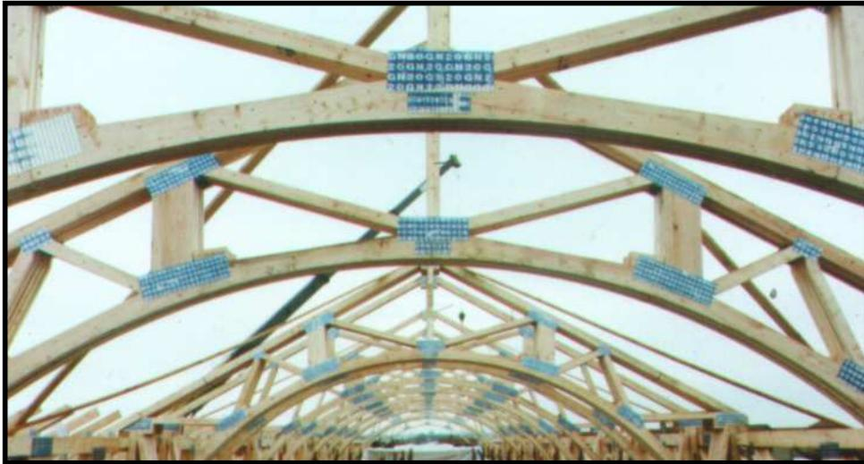
**Figure III. 19** Nail gang connections on trusses (MiTek Solutions, document on-line).
