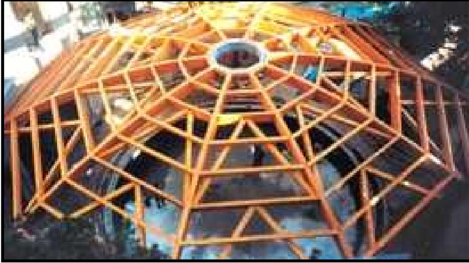
**Figure III. 35** Dome structure for the indoor swimming pool of Silyum Hotel<sup>23</sup> (Oran Mimarlık, document on-line).
