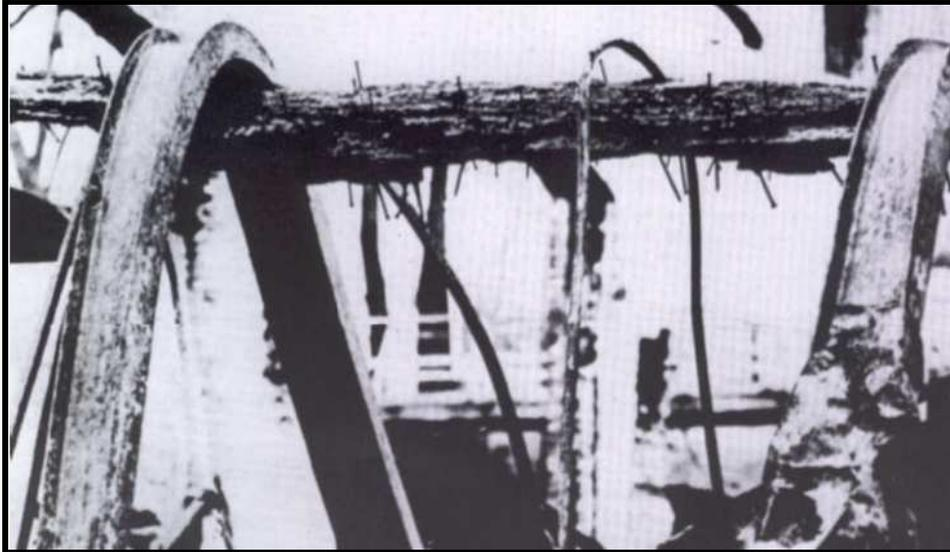
**Figure III. 31** Steel beams have melted and collapsed over charred glulam beam which, despite heavy damage, remains in place (Glued Laminated Timber Association, document on-line).
