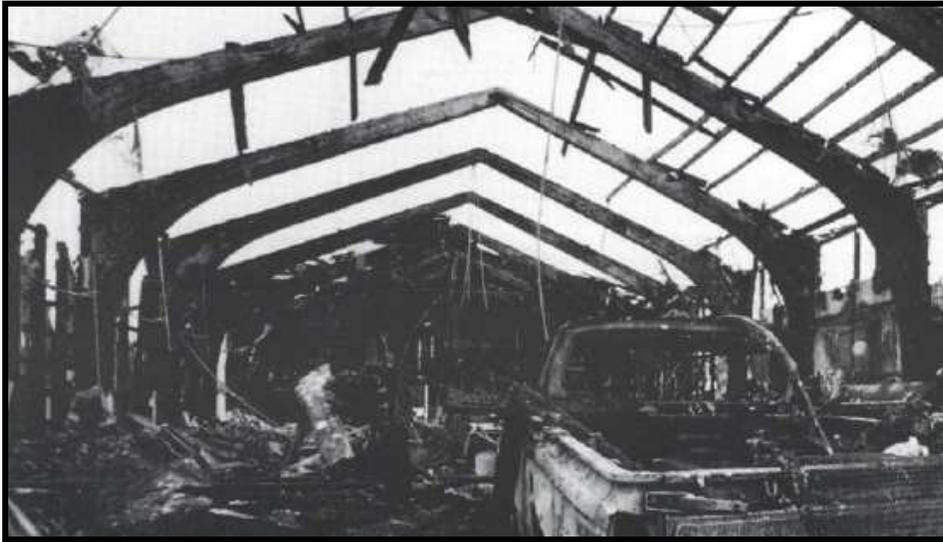
**Figure III. 29** Glulam portal frames maintained their integrity in a magnesium-fed fire. The metal walls and roof of the building melted and collapsed (Glued Laminated Timber Association Technical Data Sheet, document on-line).
