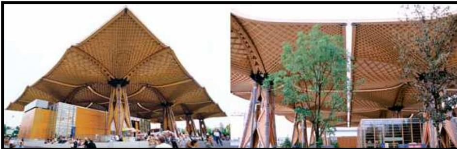
**Figure II. 54** Roof structure of the Hanover Expo Canopy; Hanover, Germany (Timber Research and Development Association, document on-line).
