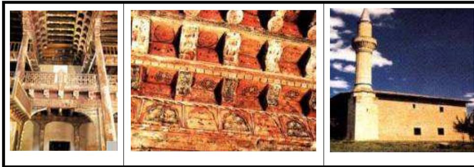
**Figure III. 39** Kasaba Mahmutbey Mosque<sup>27</sup> has a timber structure without any nail connection (Tatil Dünyası, document on-line; Kastamonu Governership, document on-line).
