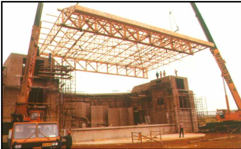
**Figure III. 11** 25 m x 30 m roof structure over theatre cantilevered off 4 support points. Structure is hold by cranes (MiTek Solutions, document on-line).
