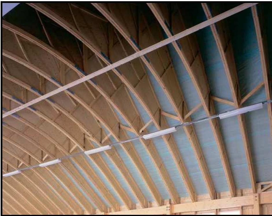
**Figure II. 23** Roof structure of Viikki Teaching and Research Farm; Viikki, Finland (Timber Research and Development Association, document on-line).
