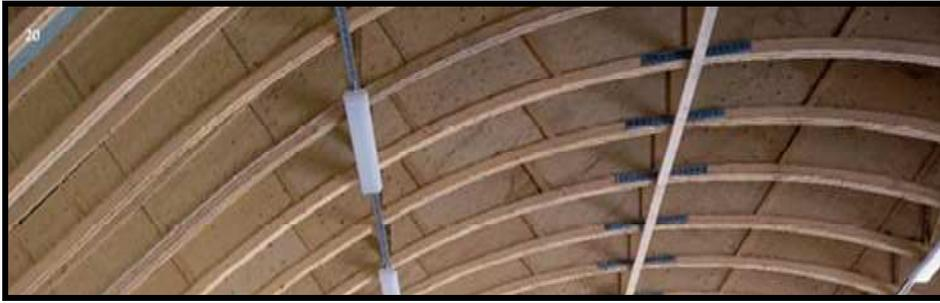
**Figure II. 22** Roof structure of Viikki Teaching and Research Farm<sup>4</sup>; Viikki, Finland (Timber Research and Development Association, document on-line).
