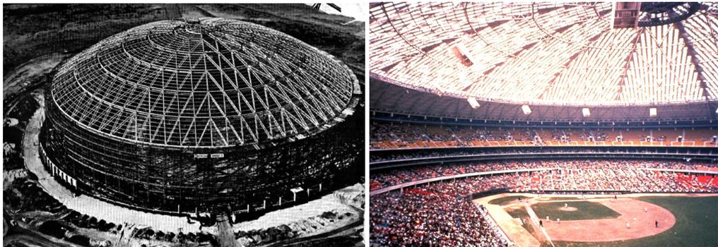
**Fig.2.7. Astrodome (Steel Lamella Dome), Houston/USA**
