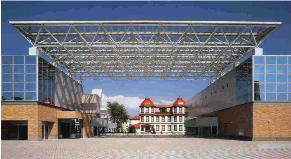
**Fig. 2.1. A Space Structure (Double-Layer Grid)**
