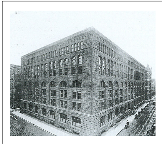
Figure II.1 Henry H Richardson's Natural Stone Façade-Marshall Field Store 1885-87 (Schittich, 2001:14).
