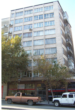
Figure III.65 Private Apartment at GMK Street No: 37 (2003)
