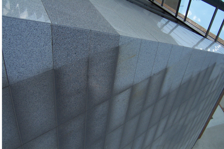
Figure III.107 Some parts of the stone panels are discolored and some are not in front of the Sport Center Pool.
