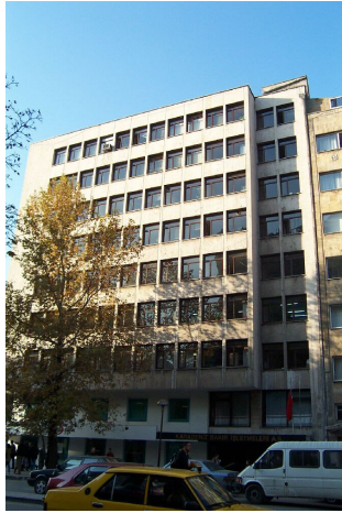
Figure III.63 Private Apartment At GMK Street No: 17 (2003)
