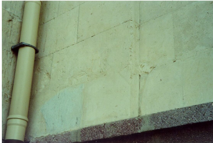
Figure III .49 Unevenness of the stone surface (2002).
