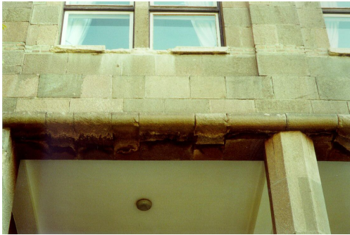
Figure III.53 a-b Deterioration of the window sill stone and discoloration of the whole stone façade caused by air pollutants (2002)
