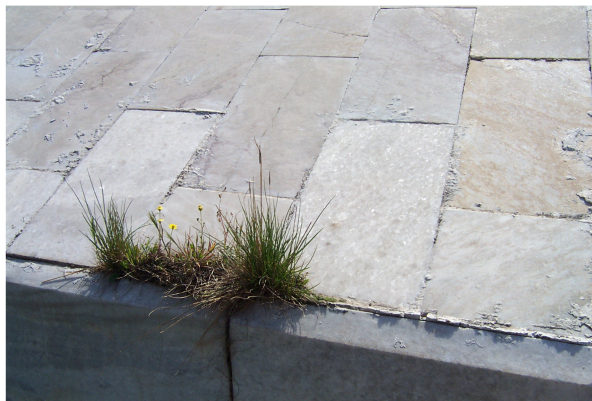
Figure III.85 Grass has grown through the joints (2004)
