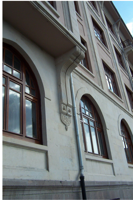
Figure III .56 a-b The surface of the decorative elements were deteriorated due to weathering and changed with the new ones during restoration. a. (2002) b.(2004)
