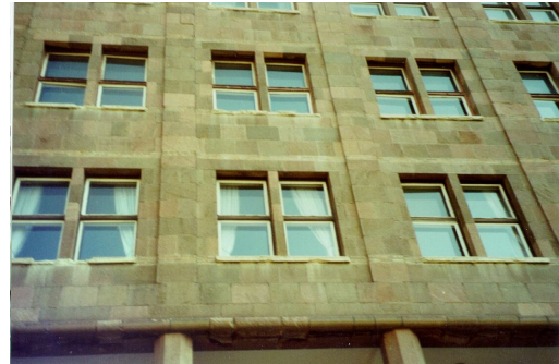
Figure III.53 a-b Deterioration of the window sill stone and discoloration of the whole stone façade caused by air pollutants (2002)
