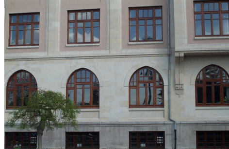
Figure III.55 a-b The arrow piece of stone panels had fallen down and replaced with a new one during restoration (2002) (2004)
