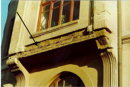
Figure III.55 a-b The arrow piece of stone panels had fallen down and replaced with a new one during restoration (2002) (2004)
