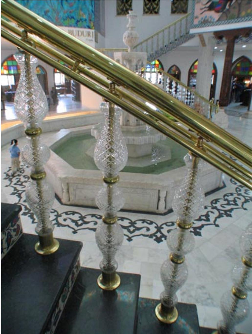
**Figure 3.31** The balustrades of the stair cases in the atrium space are made of crystal. These balustrades are the imitation of the ones in the Dolmabahçe Palace in İstanbul.
